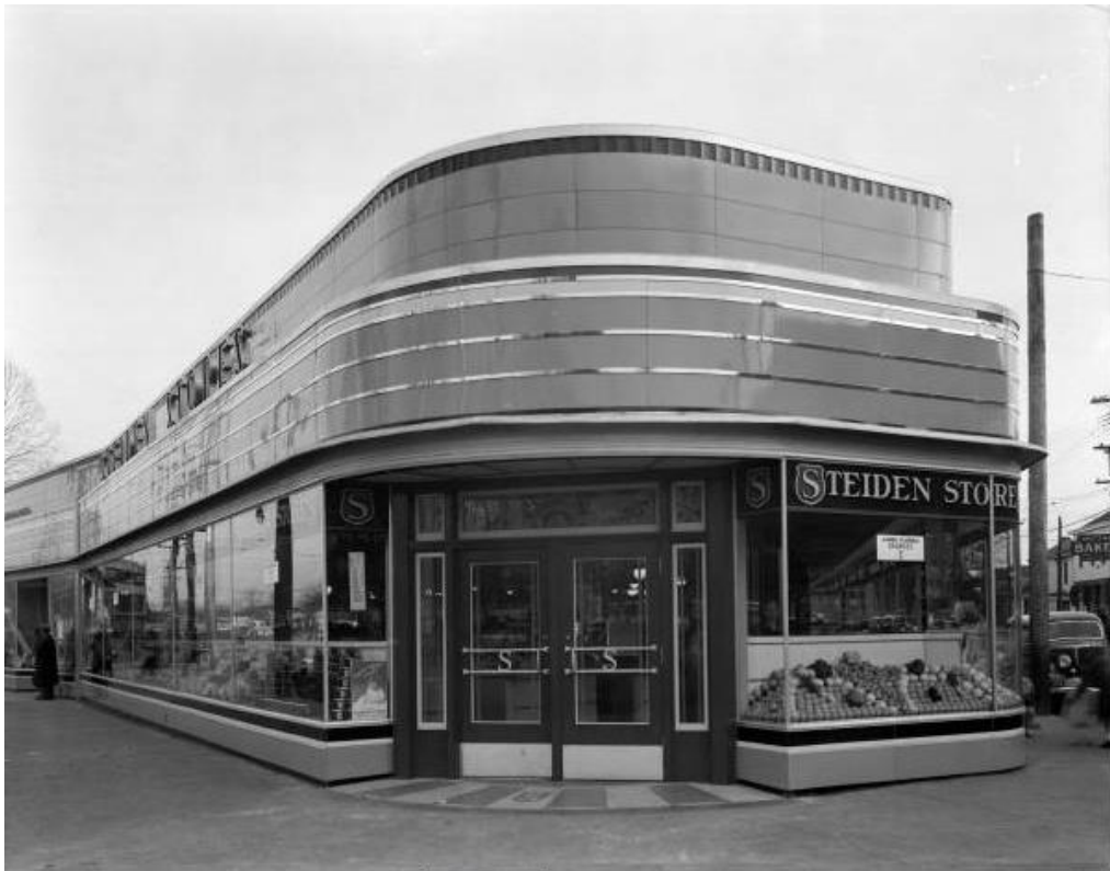
Steiden Store (Bardstown Rd—now demolished)
