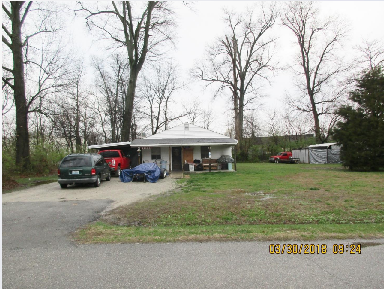
Across Street to North
