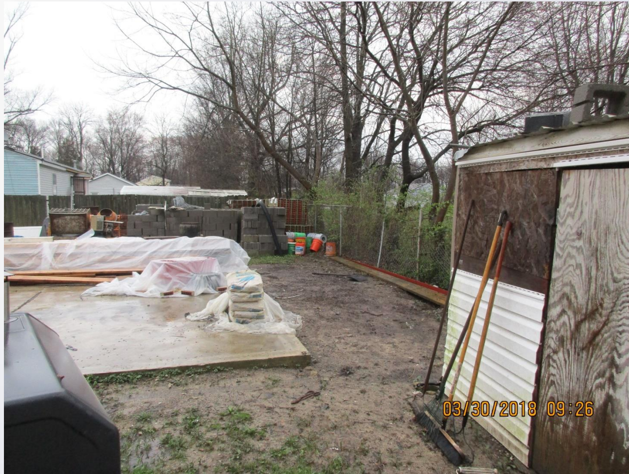
Existing Slab Foundation
