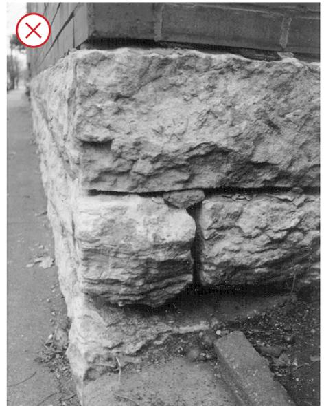
Repoint a deteriorated masonry joint. Utilize a mortar mix that is compatible with historic masonry and that will allow moisture to escape.
