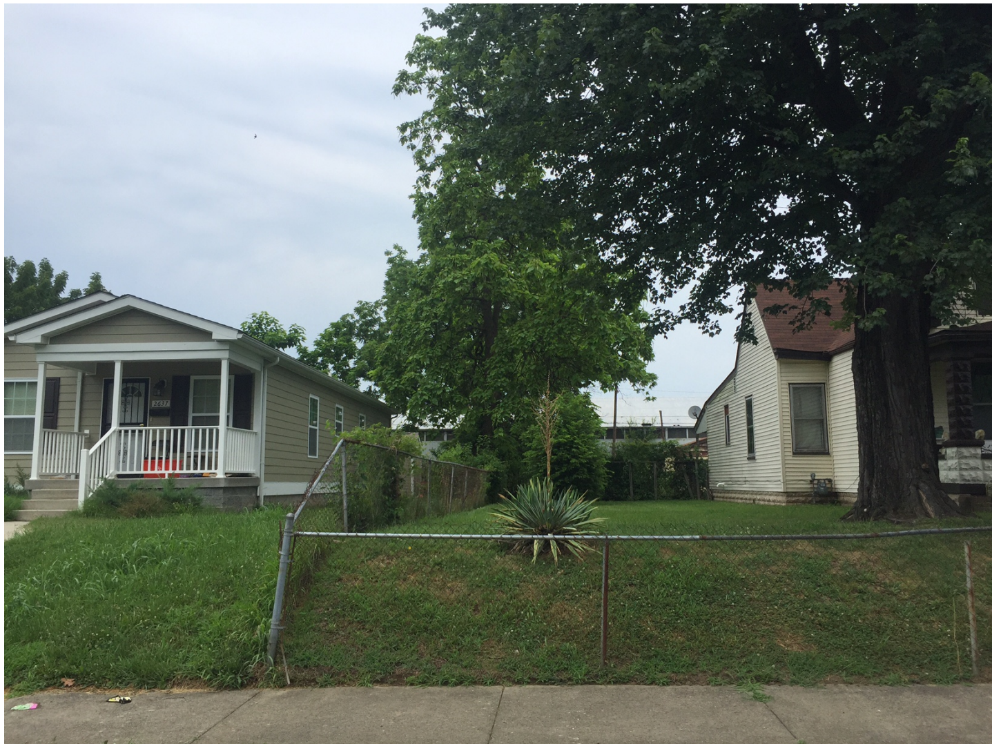
Front view-2635 Garland Ave
