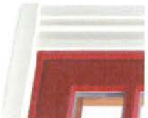
3/4" backboard and bead casing and 1 1/2" sill nose shown on casement
