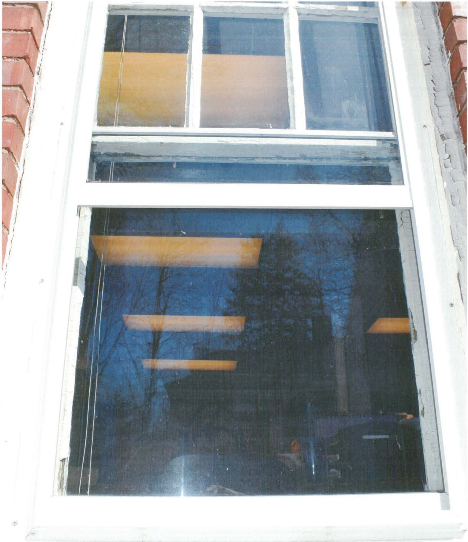
2427 Glenmary Ave. Lower School West Elevation
