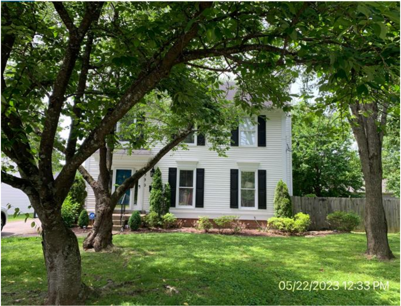
Front of subject property.
