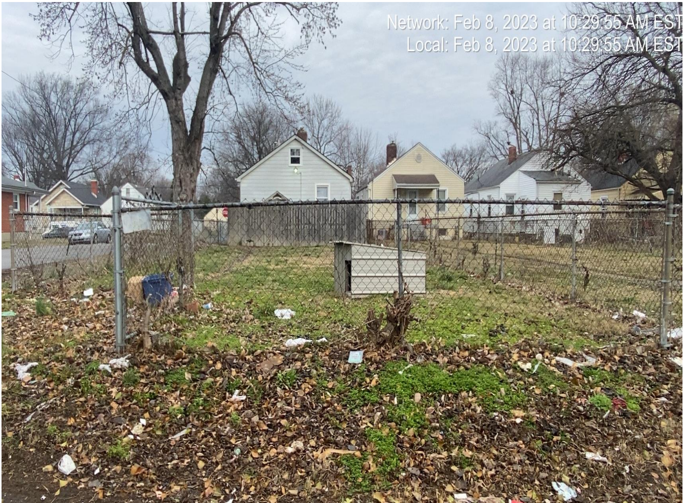
Rear of subject property.
