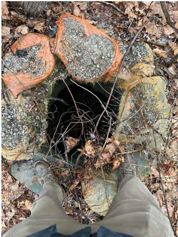
Northeastern Storm Sewer
