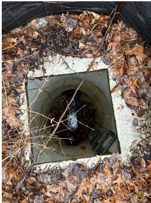
Northeastern Storm Sewer
