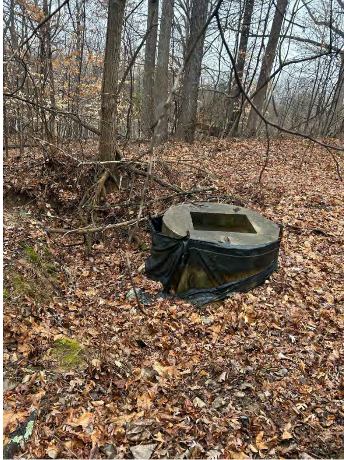
Southern Storm Sewer
