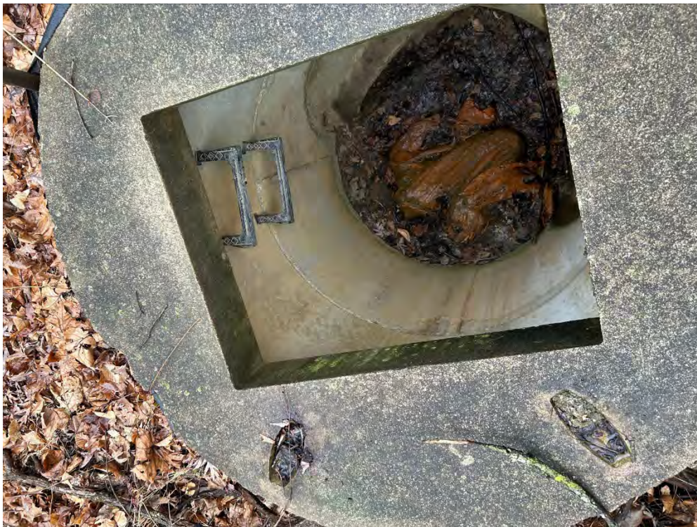
Southern Storm Sewer
