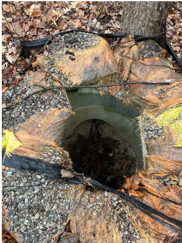
Southern Storm Sewer
