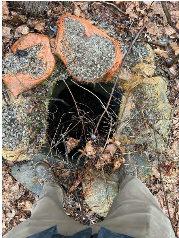
Northeastern Storm Sewer
