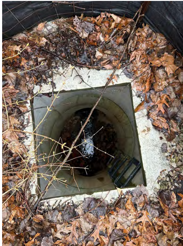
Northeastern Storm Sewer
