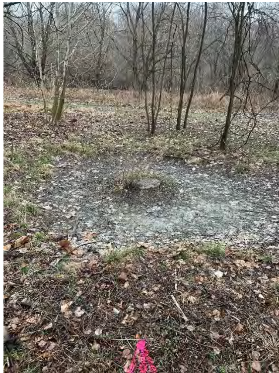
North Central Sanitary Sewer
