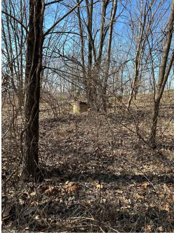
South Central Sanitary Sewer
