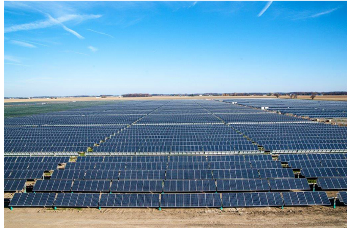
20 MW solar field in Bowling Green, Ohio produces approximately 40,000 MWh of electricity on 165 acres
