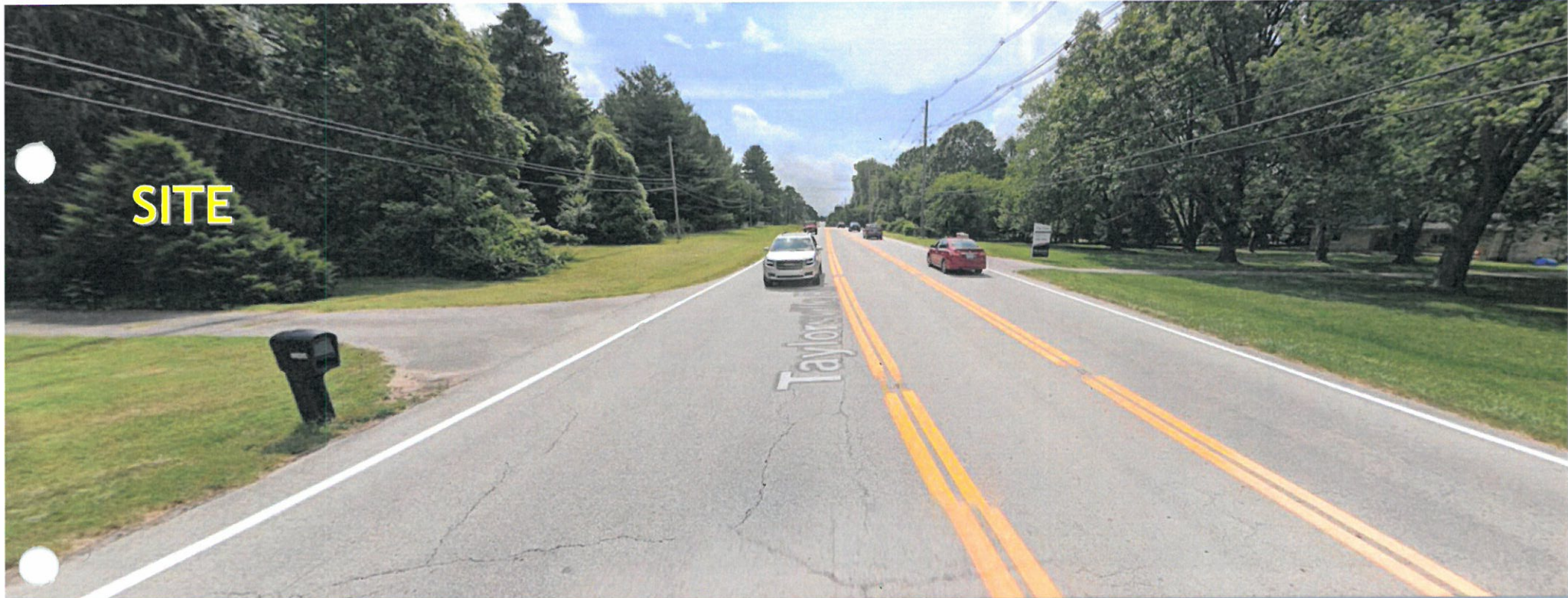
View of Taylorsville Road looking west. Site is to the left.
