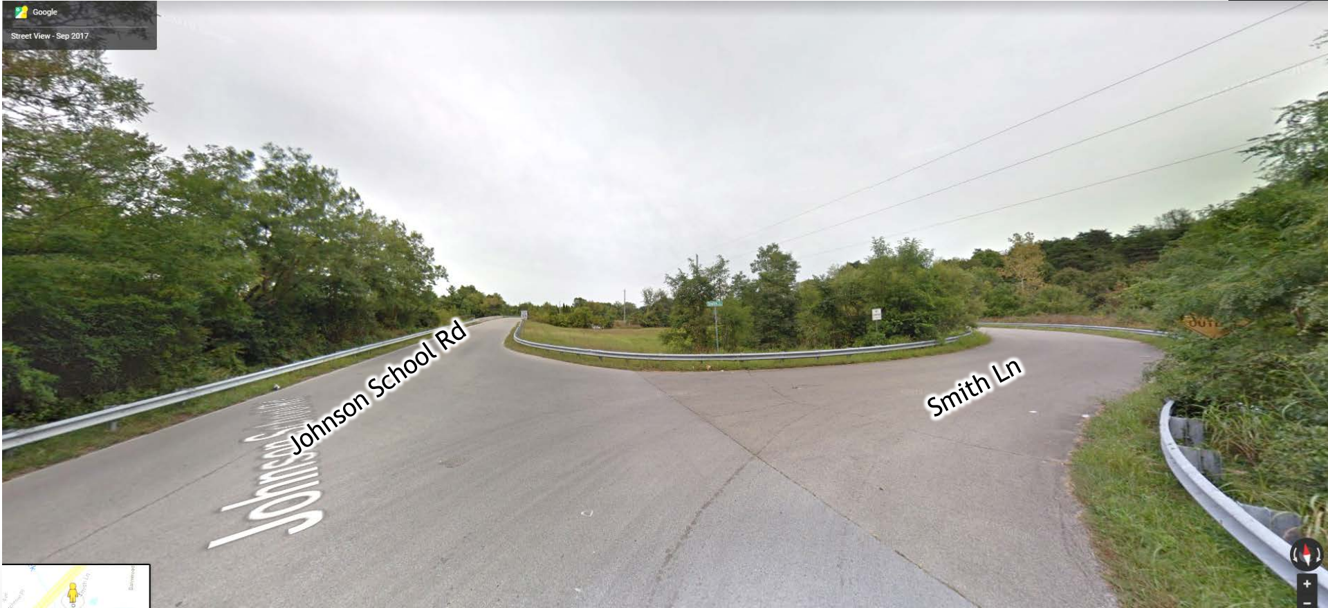
Looking north towards intersection of Johnson School Rd and Smith Lane
