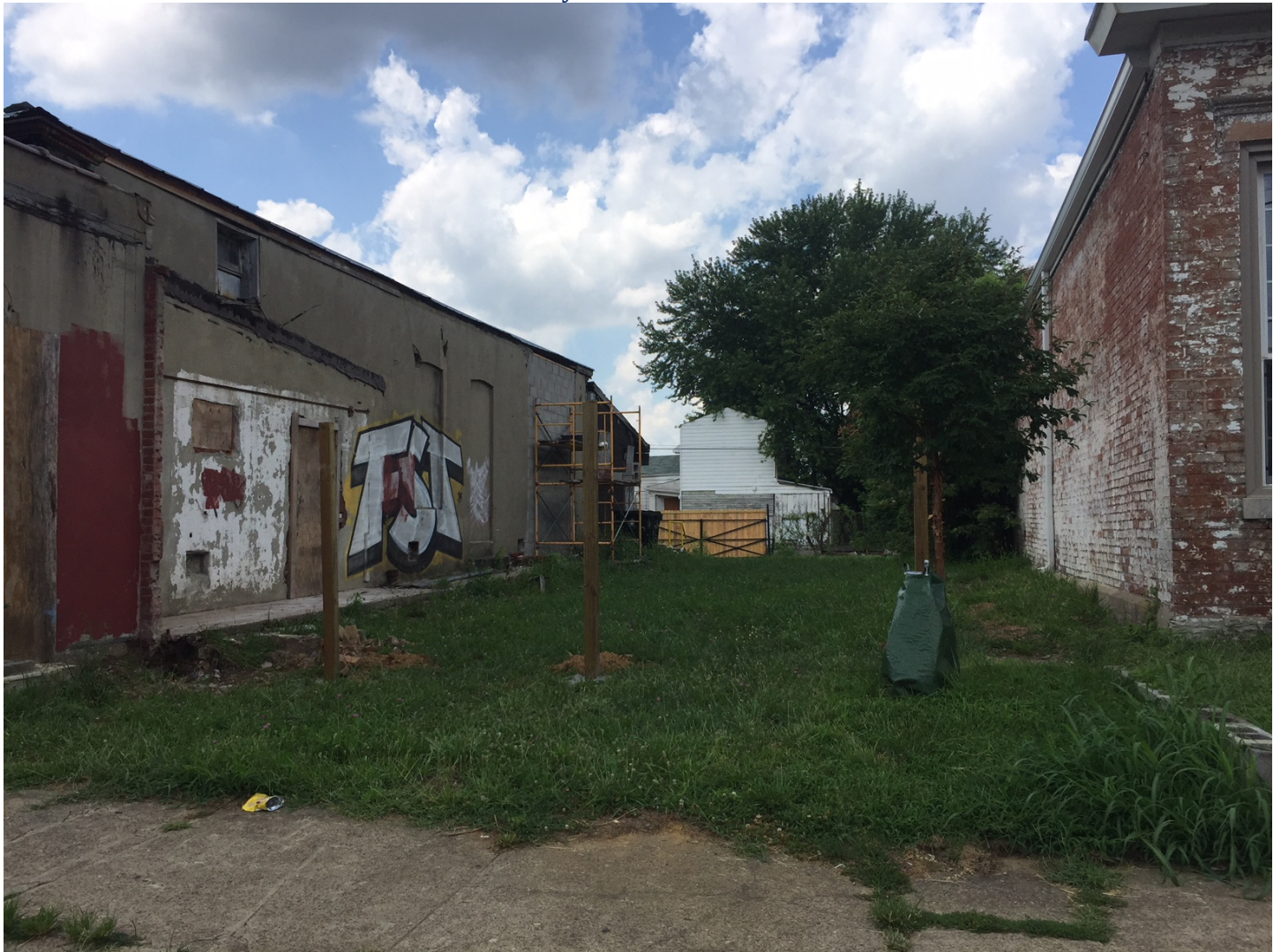
South Shelby Street – Front View
