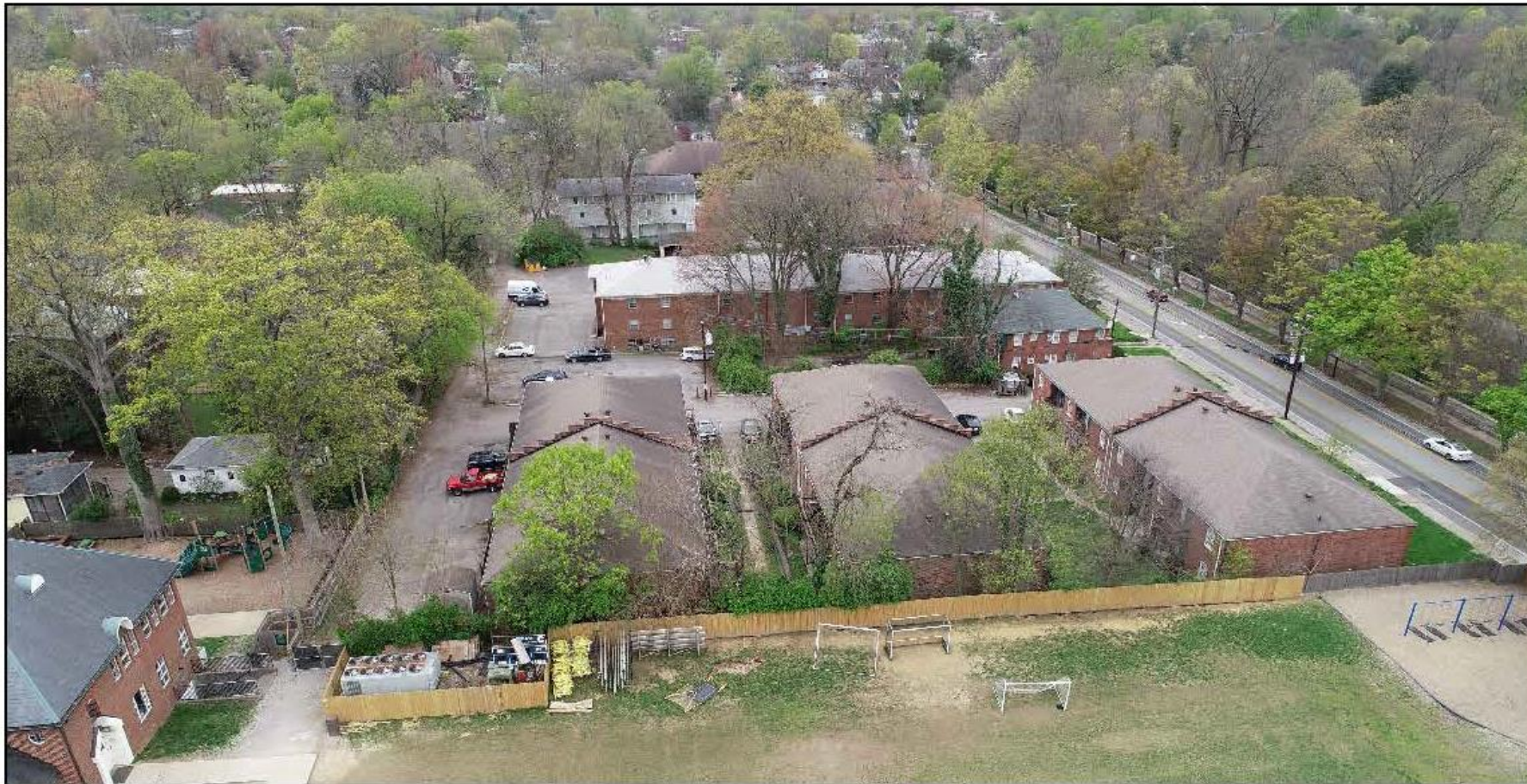
YORKTOWN TO THE NORTHWEST - YORKTOWN APARTMENTS TO BE DEMOLISHED
