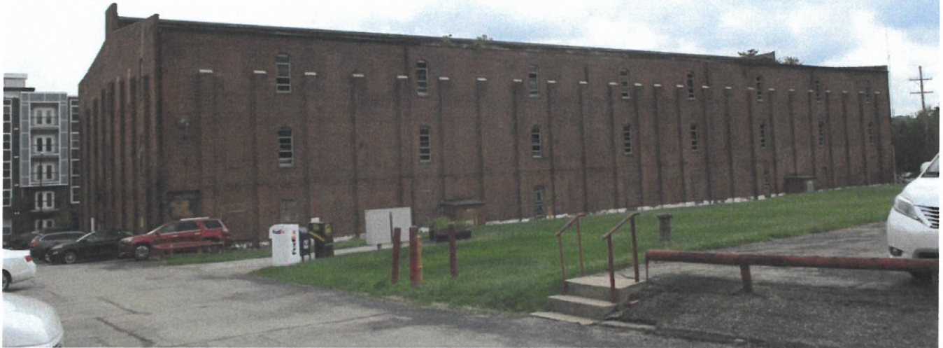
100 Distillery Commons Looking Northeast
