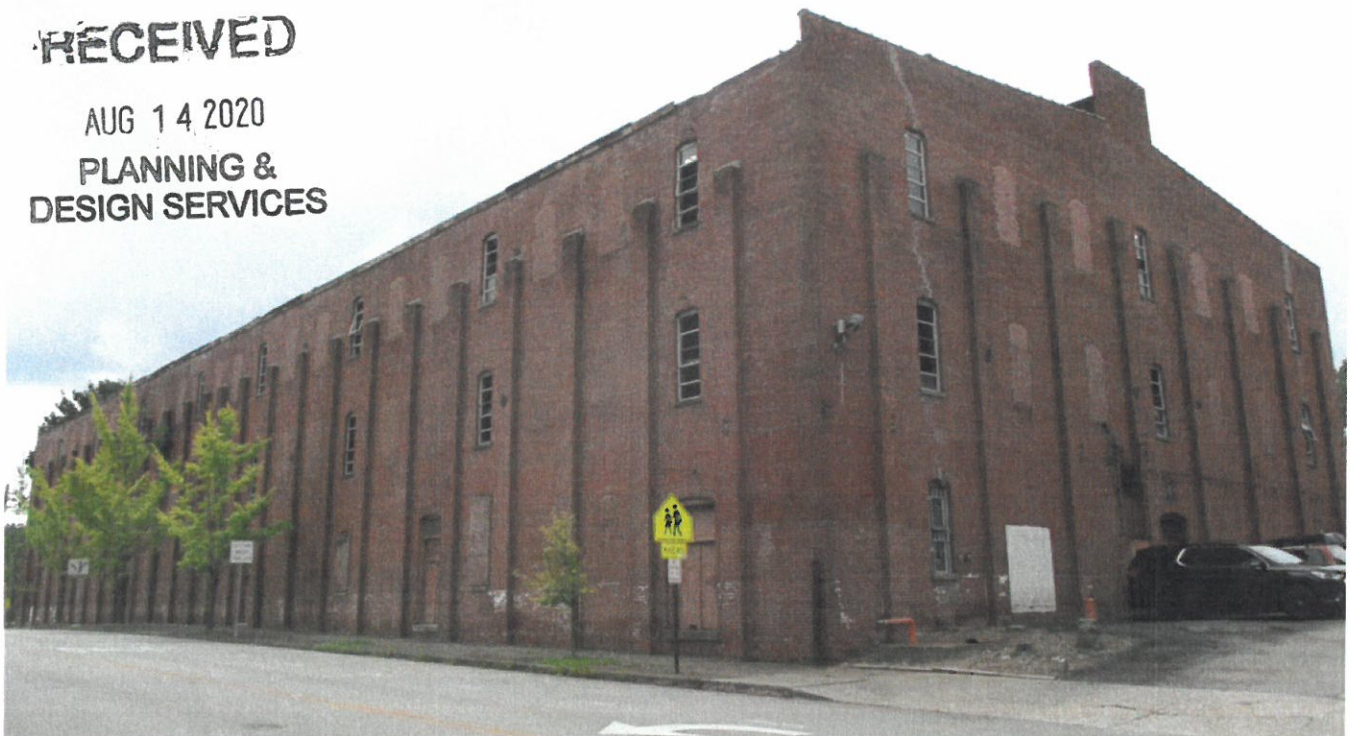
100 Distillery Commons Looking Southeast
