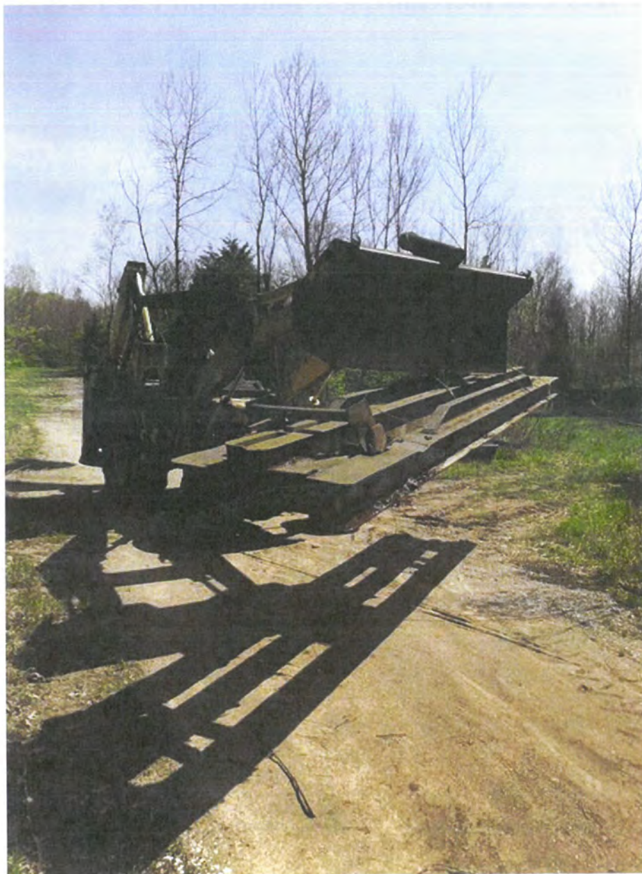
2014 - Loading house moving steel to head to job site.
