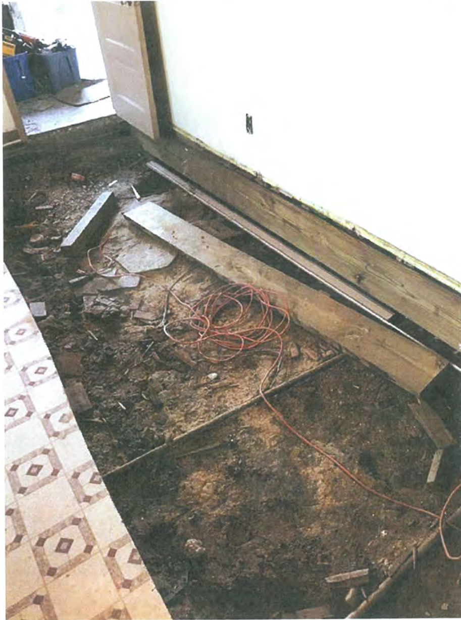
2018 - Repairing and replace failed floor joists.
