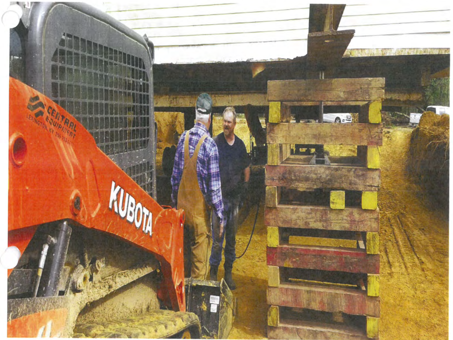
2019 - Visiting job site where rented steel is being used.
