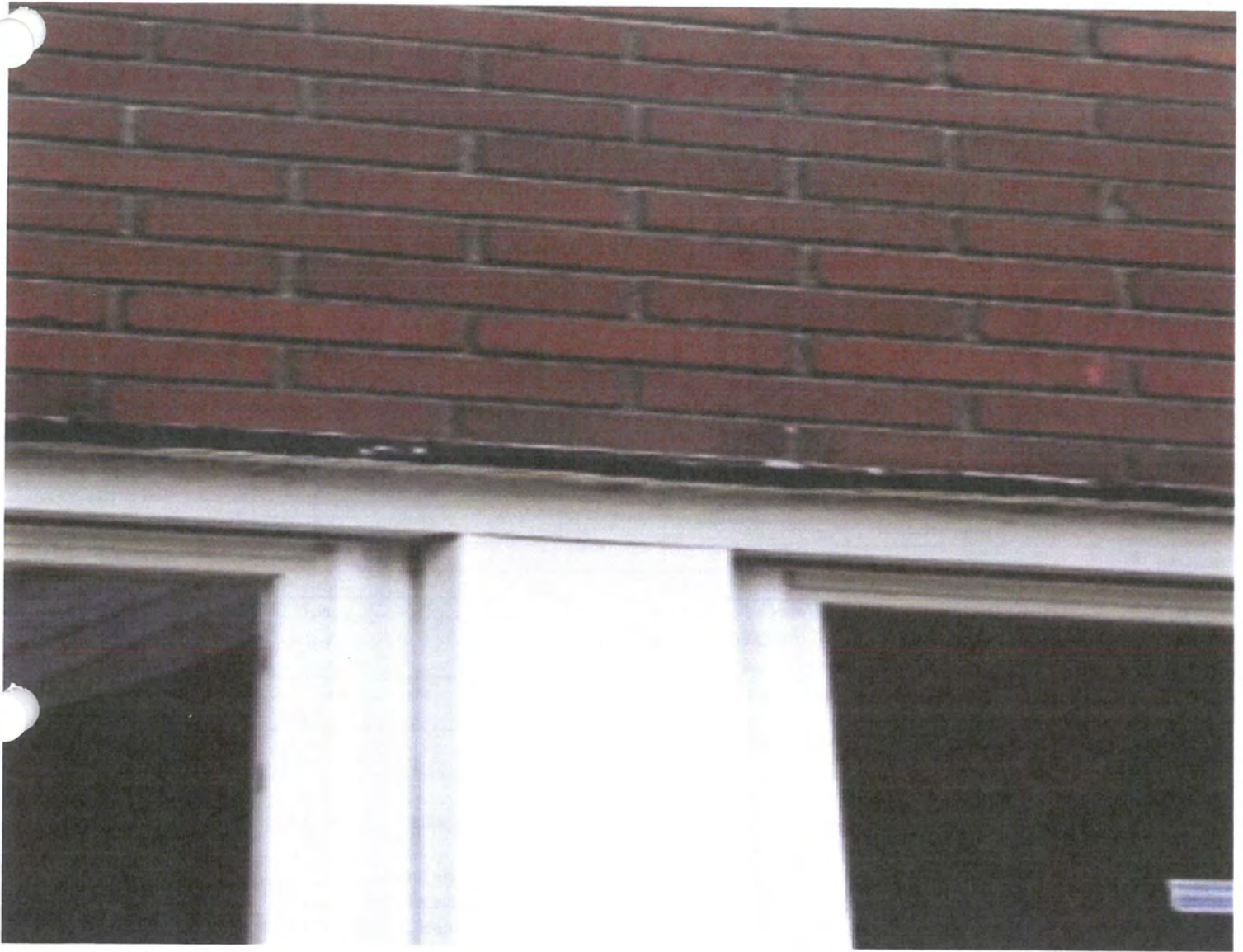
2011 - Foundation repair - jacking up brick to level.
