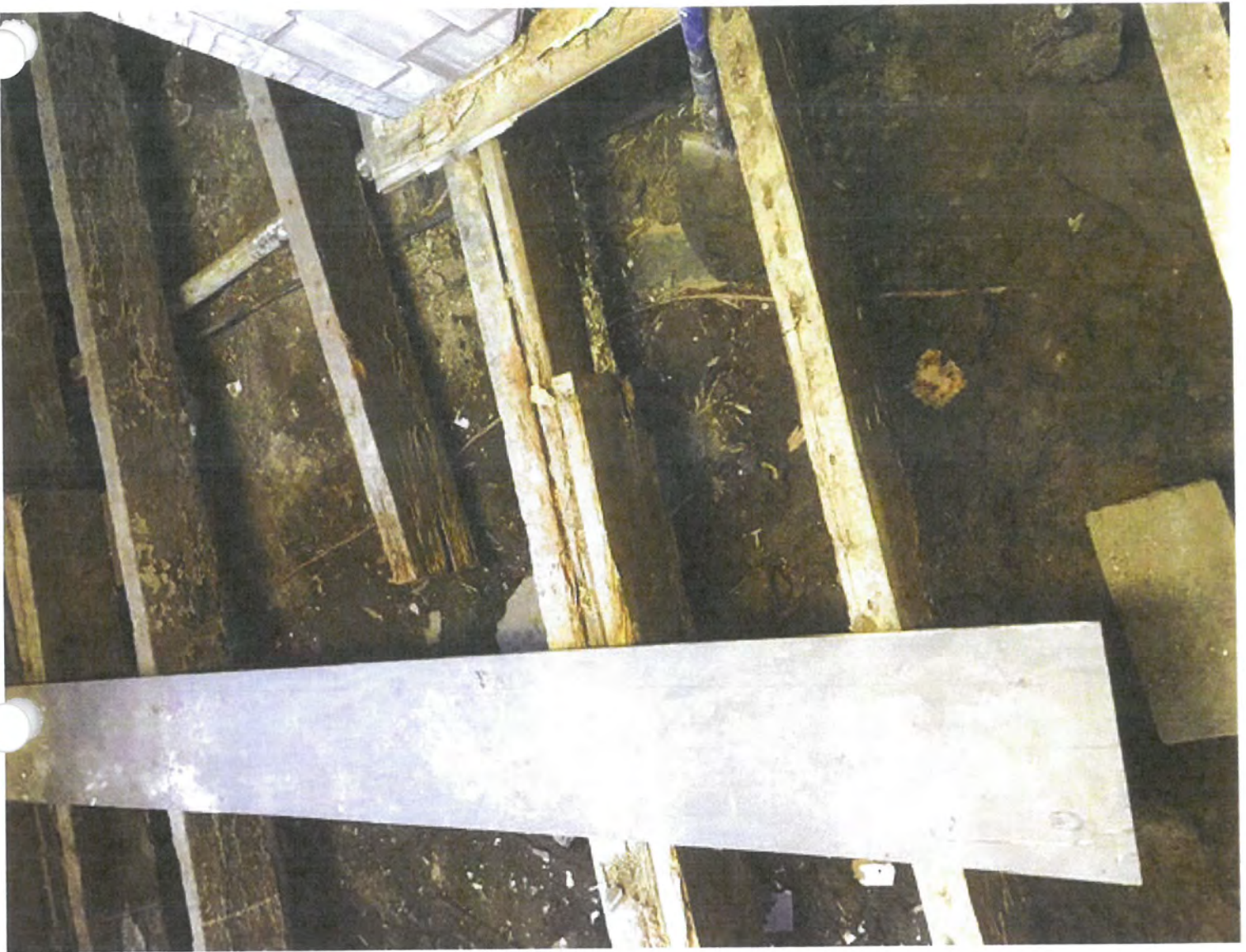
2013 - Jacking up house and leveling and replacing failed floor joists.
