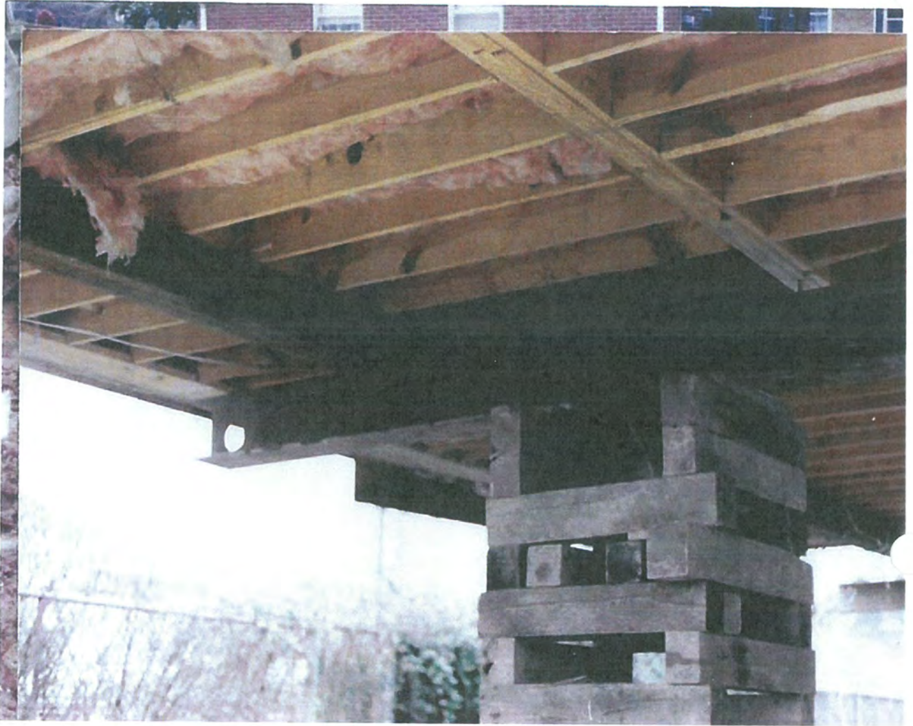
2010 - House moving job, house on cribs 12 feet high.
