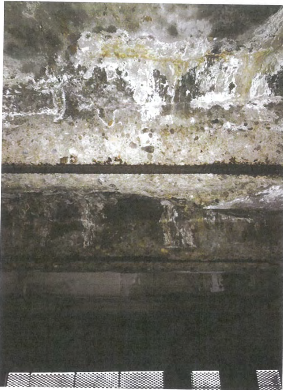
2015 - Multi level parking garage with structural and concrete surfacing repairs.
