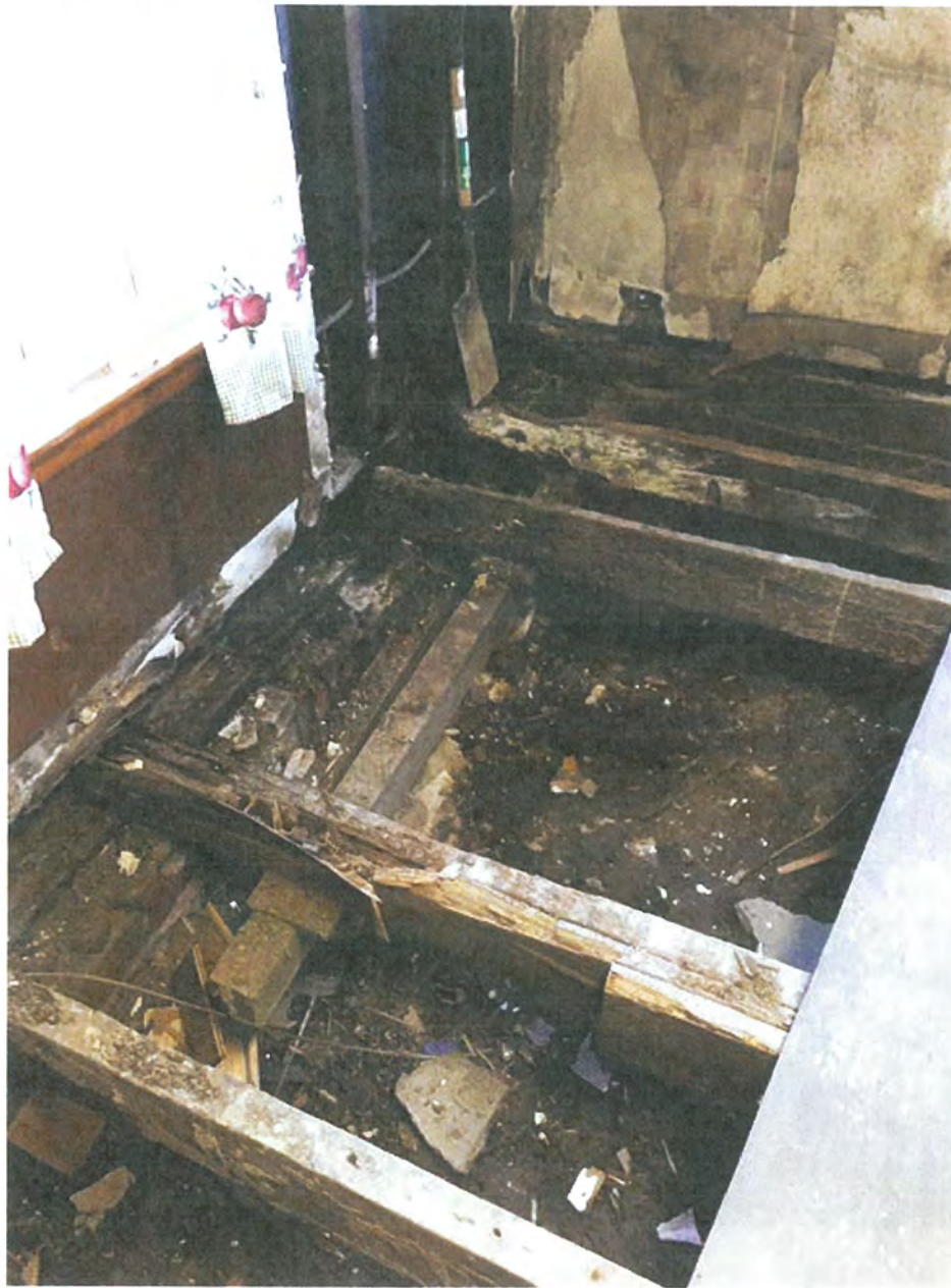
2013 - Jacking up house and leveling and replacing failed floor joists.
