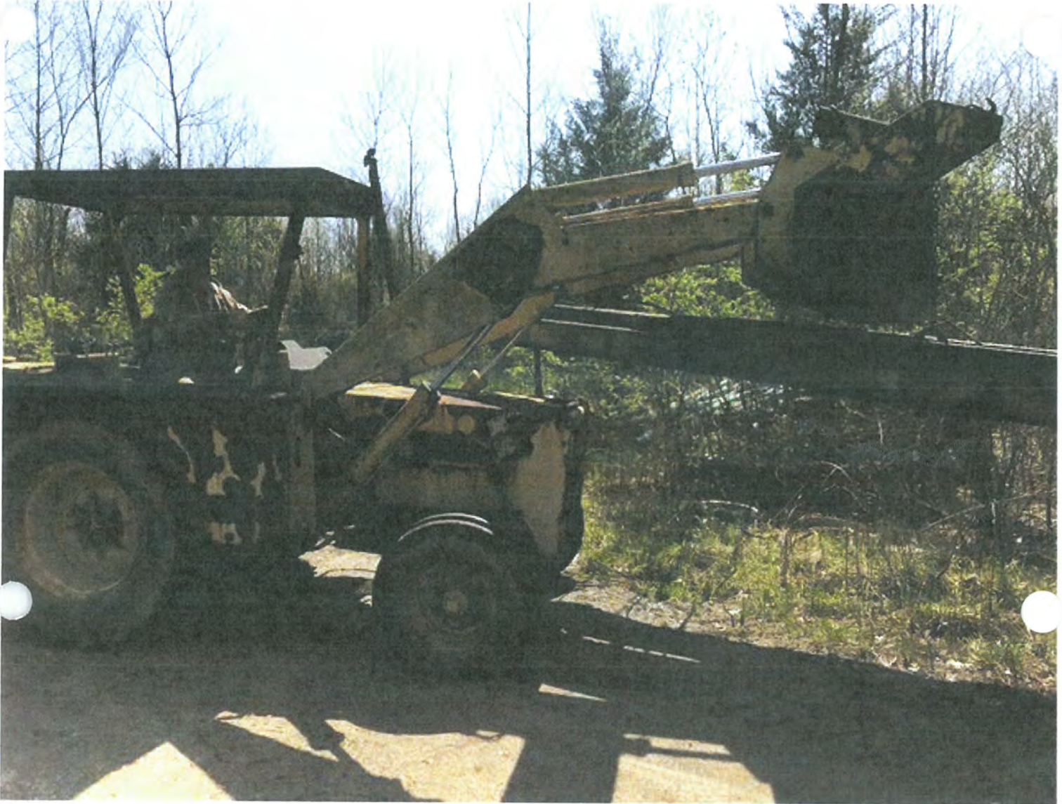
2014 - Loading house moving steel to head to a job site.
