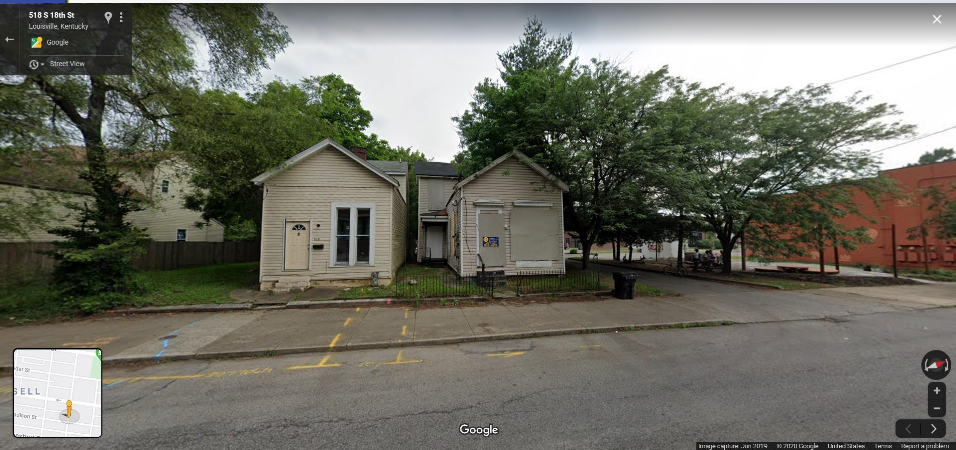
View of site from S 18 th Street
