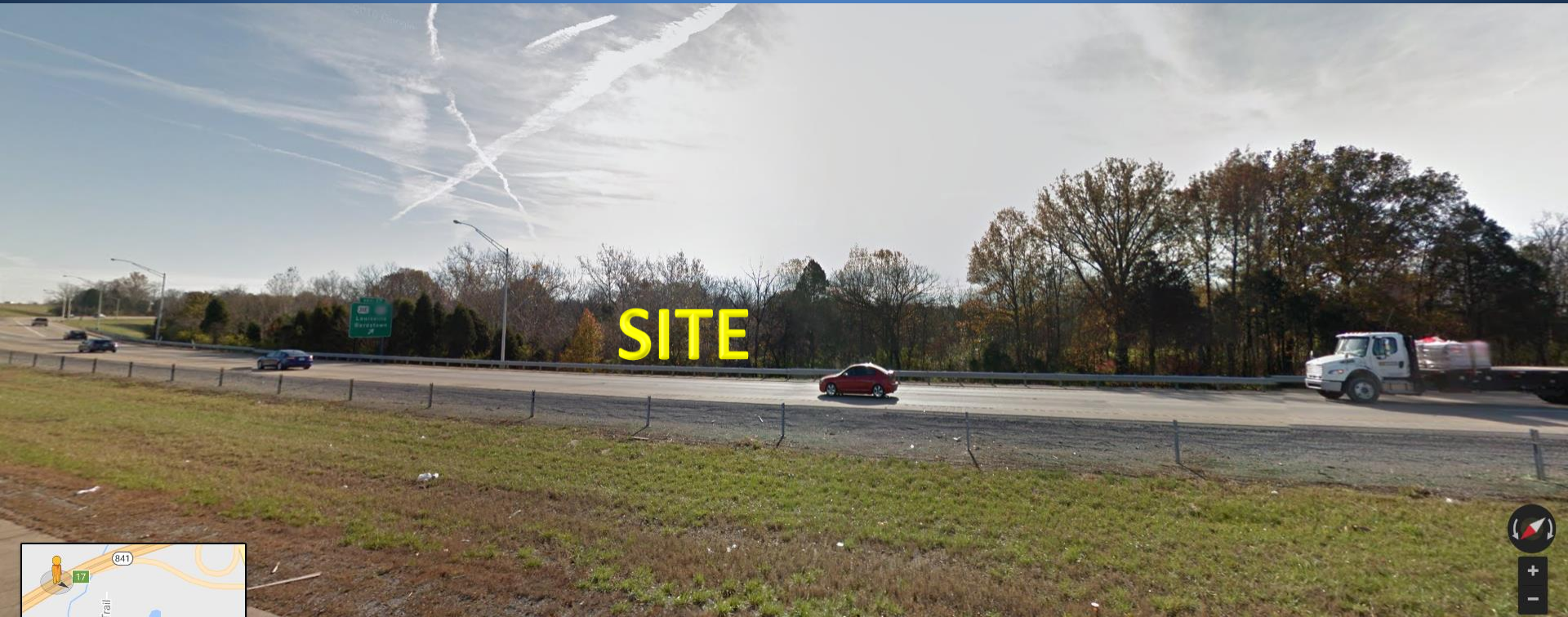
View of site from Gene Snyder Freeway.
