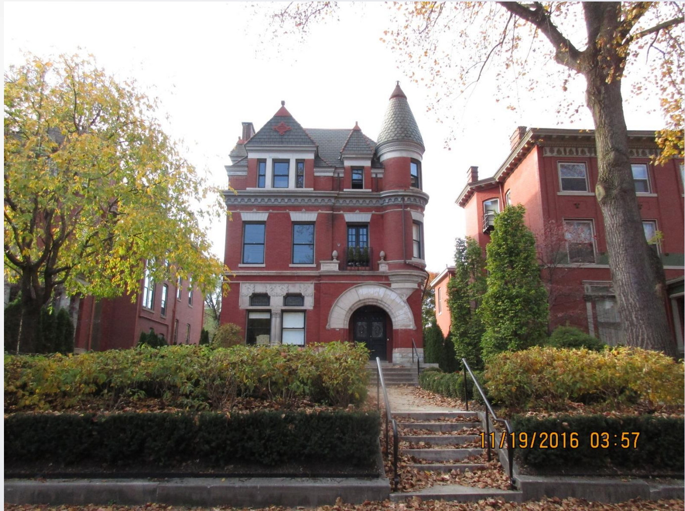
Looking at the principal structure from Third Street.
