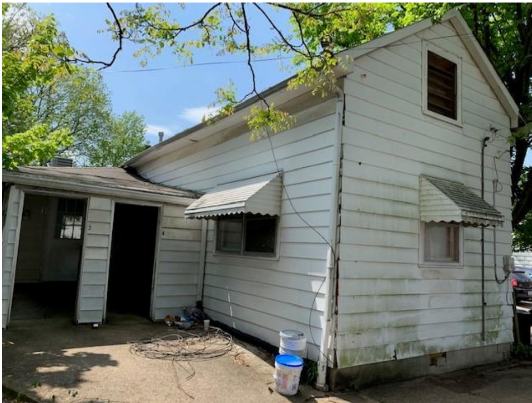
Rear elevation Staff photo
