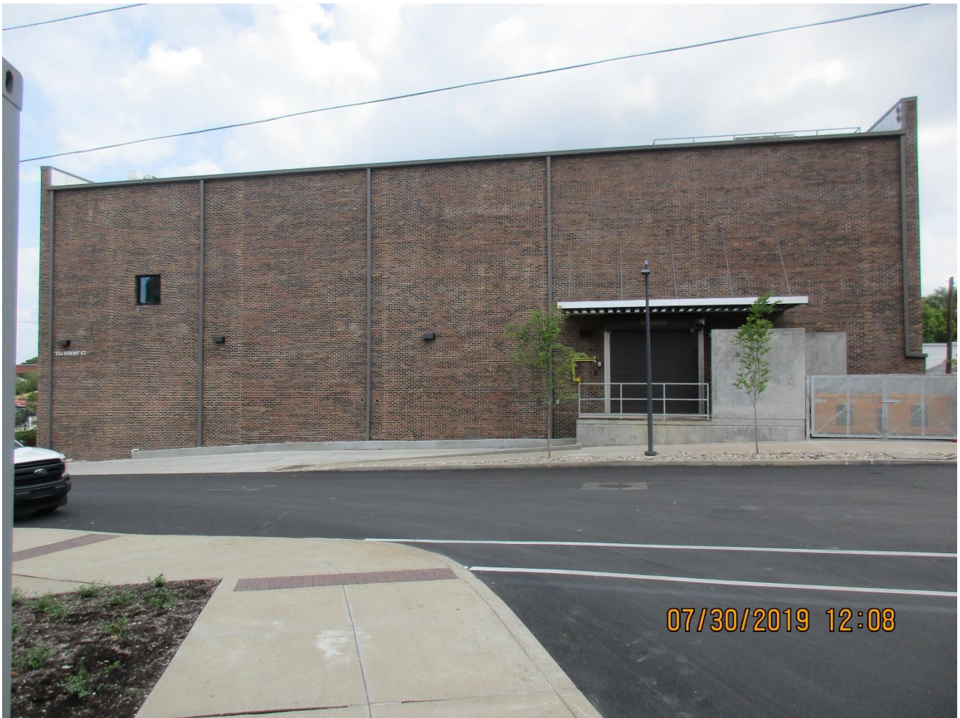
Façade of the proposed sign location.
