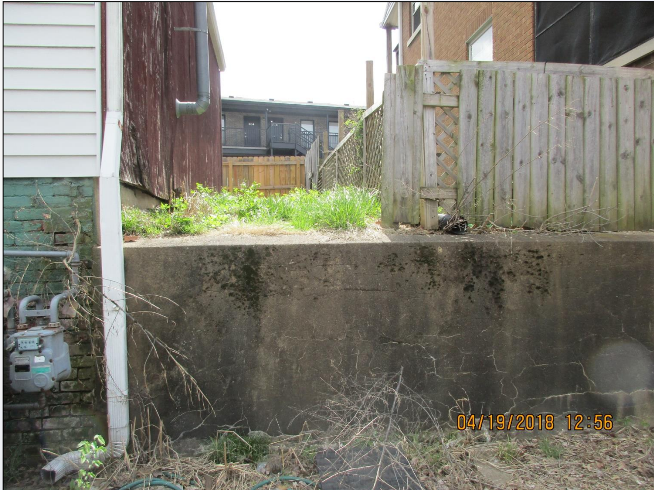
The elevated rear yard.
