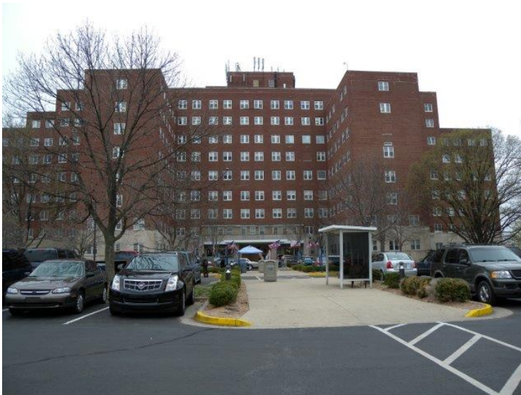
Main Hospital, main façade, northeast side
