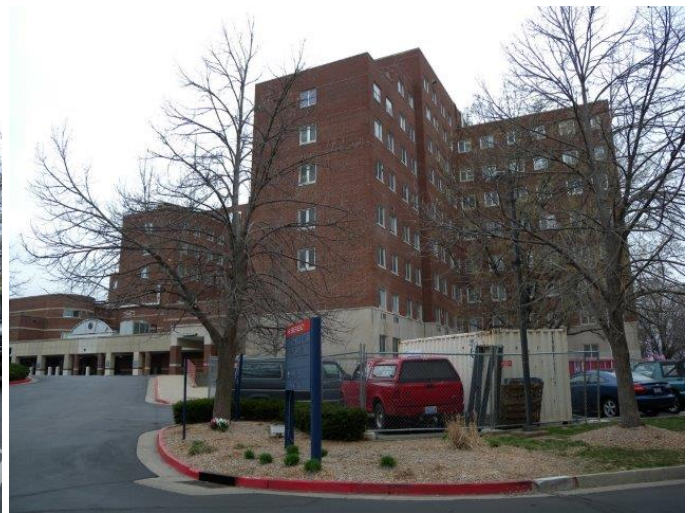
Main Hospital, East facade
