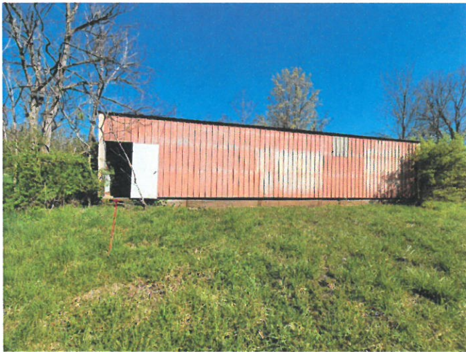
Photo 57 – View of remnant shed
