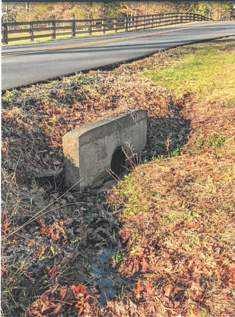
Headwall 2 – North Side
