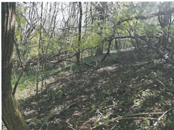
View of slope head (Northeastern Portion).
