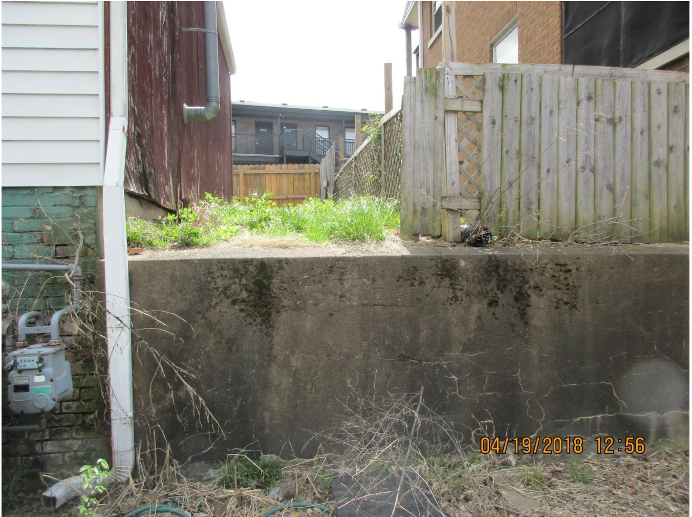
The existing rear yard as seen from the Lucia Avenue sidewalk.
