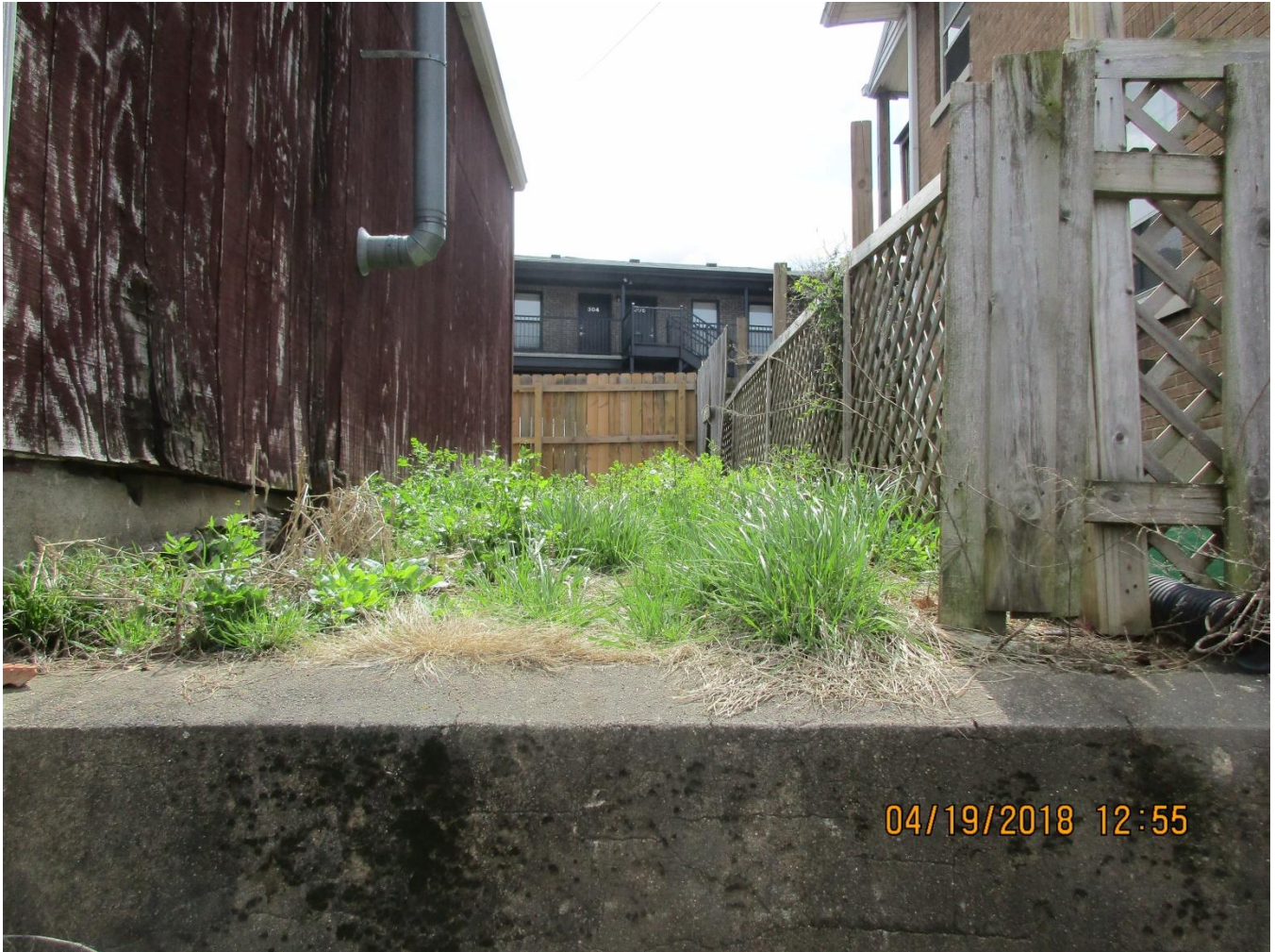
The existing rear yard is elevated from grade.
