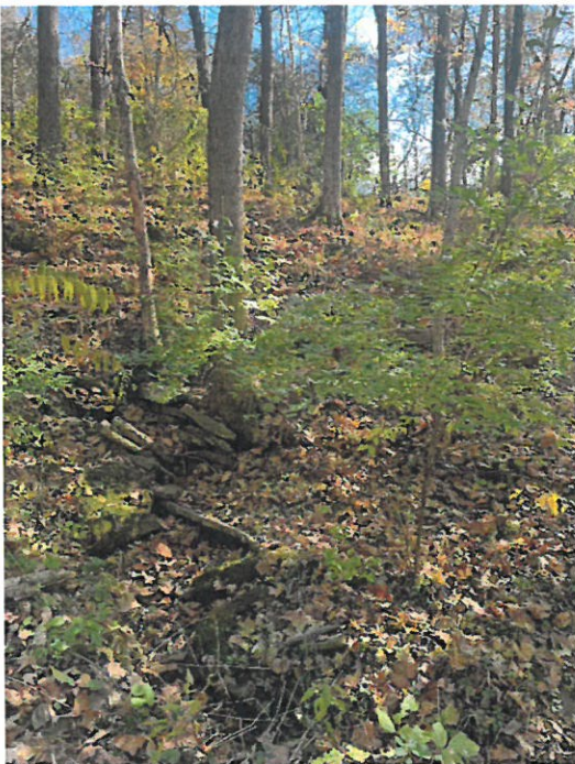
Area 8: Rock Outcropping, Minor Instability
