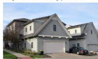
Carriage House with unit accessed off a back yard
