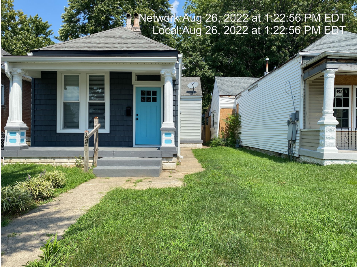
Left of subject property.
