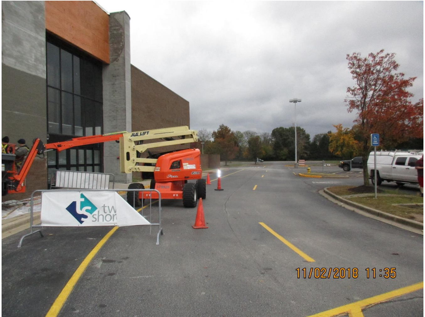
Looking northeast toward parking lot.
