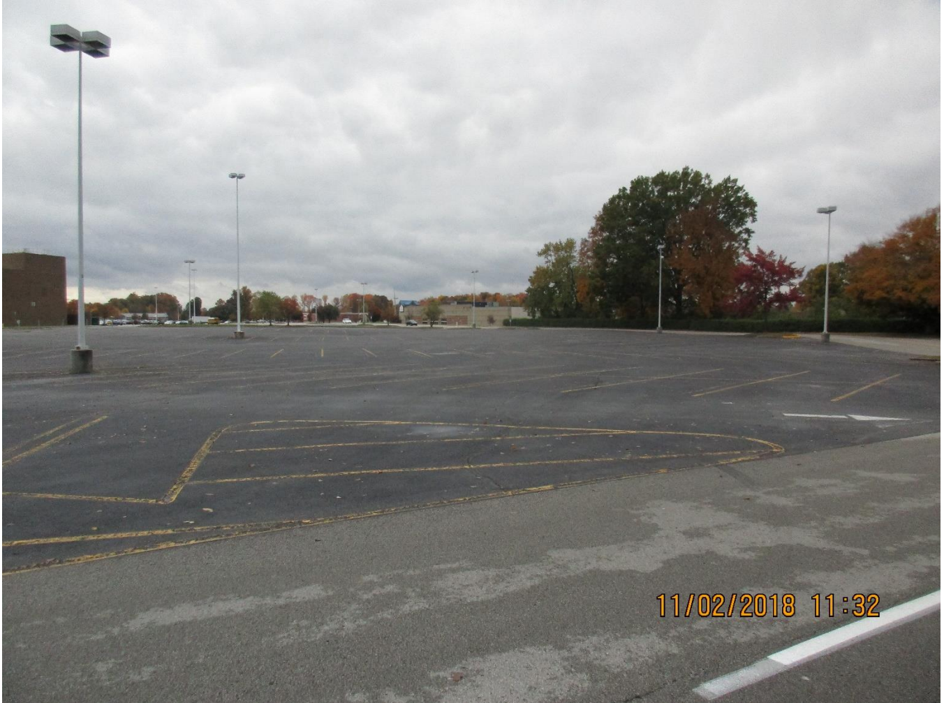
Looking west from rear of parking lot.
