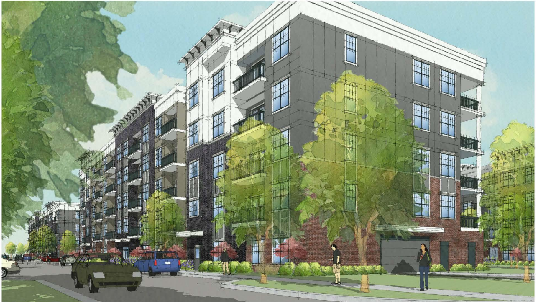
56 Residence Building - Internal View
