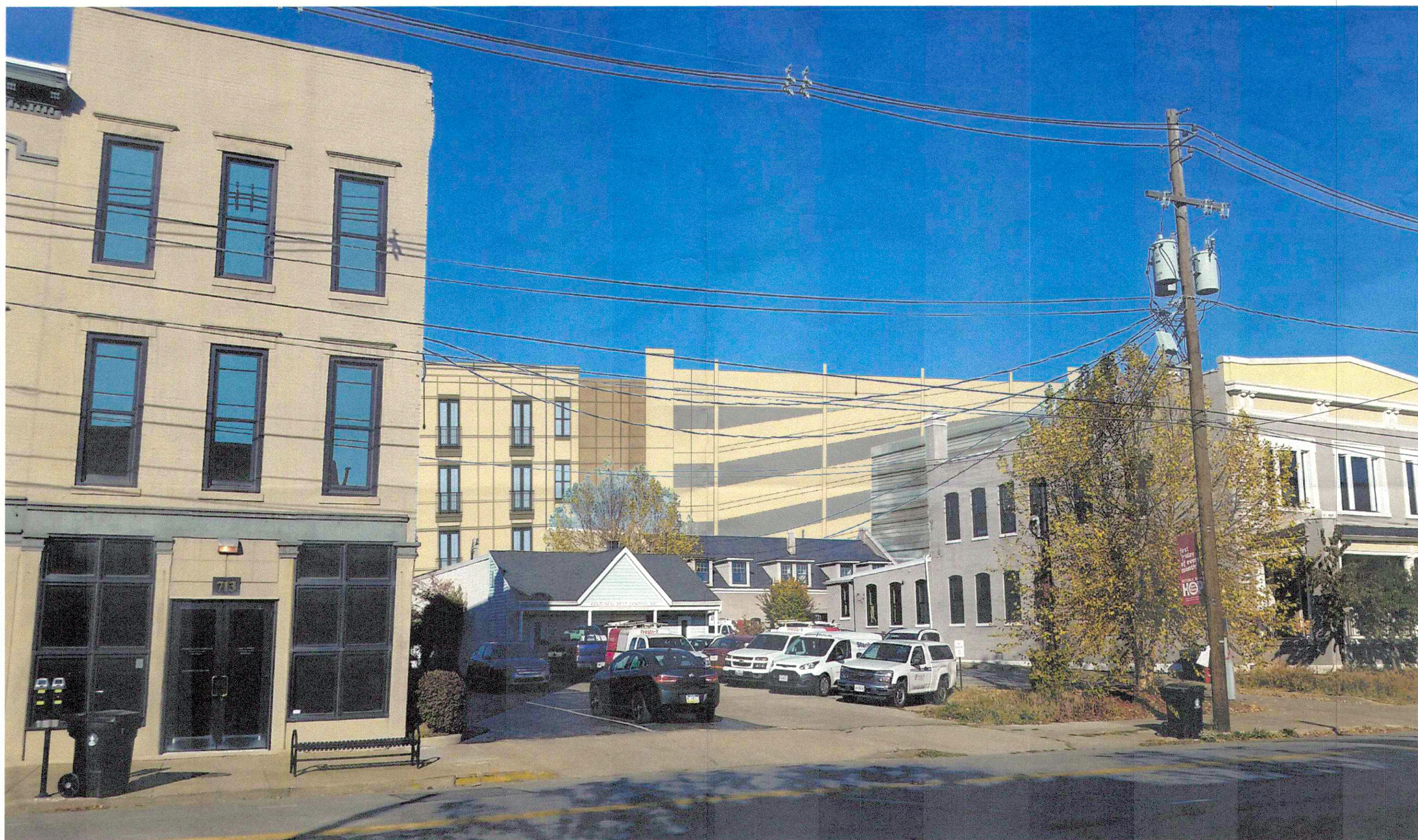
VIEW NORTHEAST FROM MARKET STREET - AFTER
