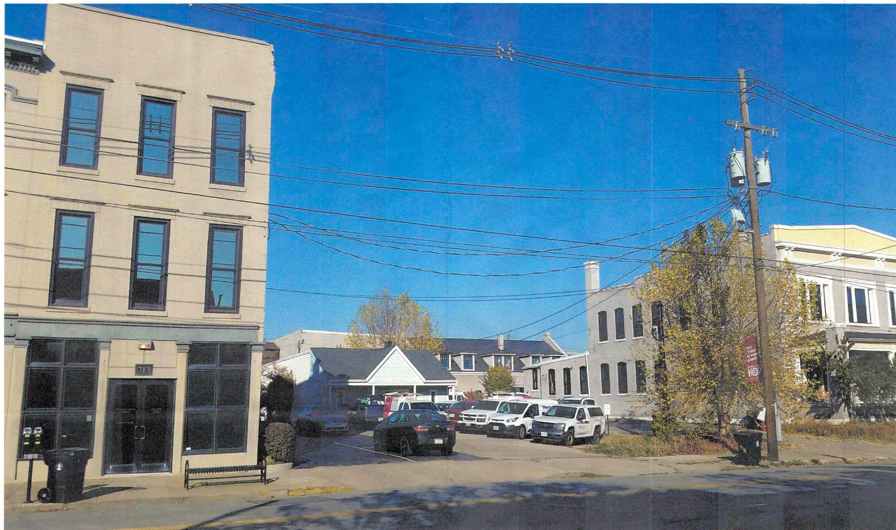
VIEW NORTHEAST FROM MARKET STREET - BEFORE
