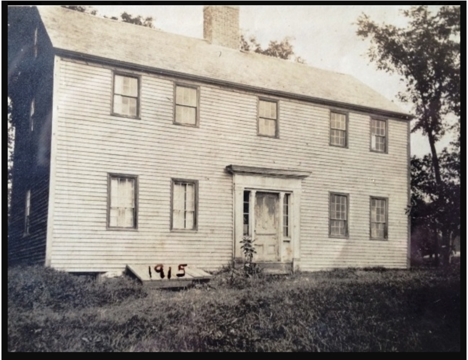
Bray House, Kittery Point, Maine
