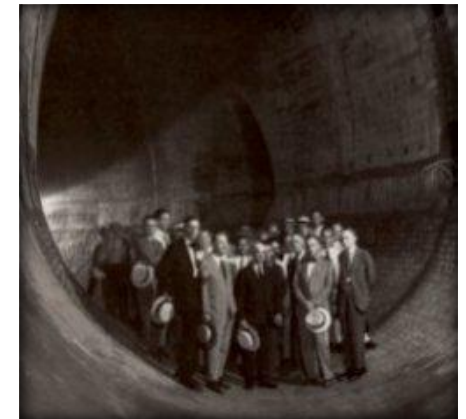
The Southwestern Outfall was completed in the early 1930s. Courtesy of the University of Louisville Photo Archives
