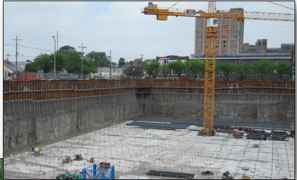
Logan St Basin Construction
