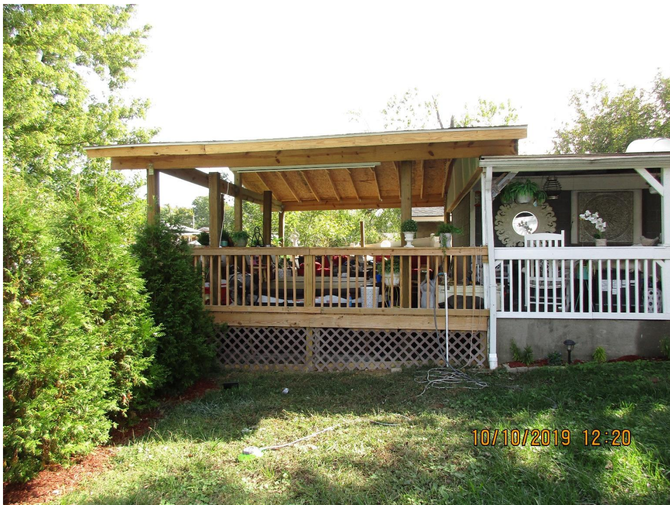
New deck attached to existing garage.
