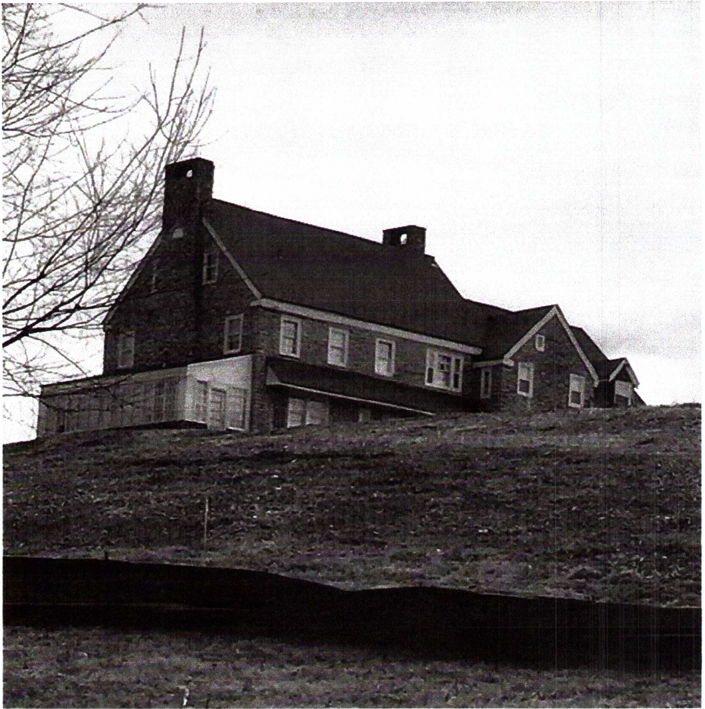
Photo #2 South + West Sides; Taken from Blankenbaker Lane
