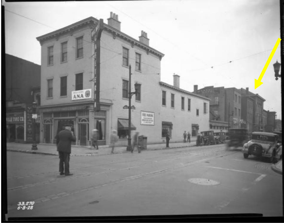
Figure 13. 1928 Metropolitan Sewer District Photograph of S. Third St and W. Walnut, looking east. Liberty Hall is on the far right side of the photograph.
