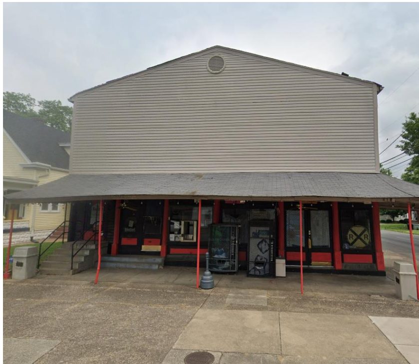
Figure 24. Klondike Hall, 2201 Garland Ave.
