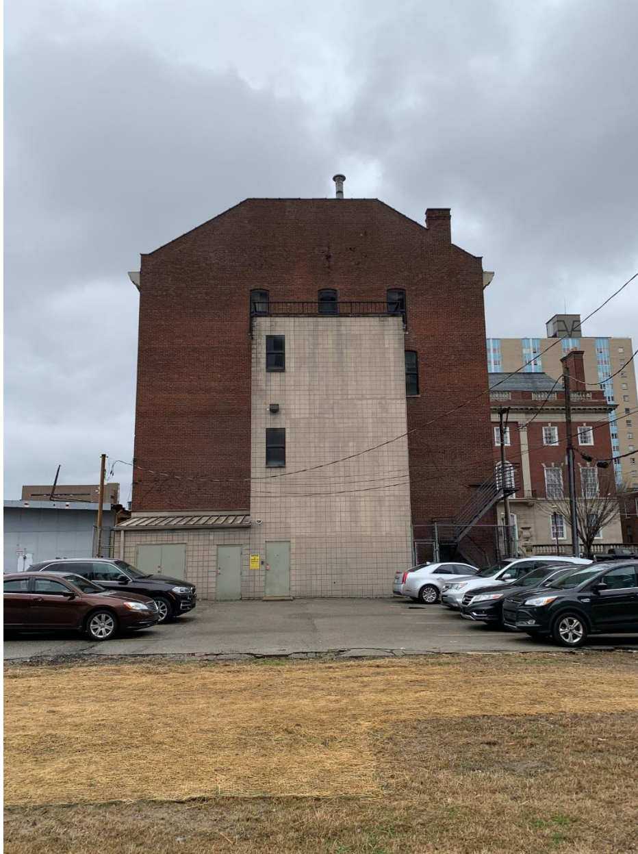
Figure 5. View looking at South at the North (rear) elevation.
