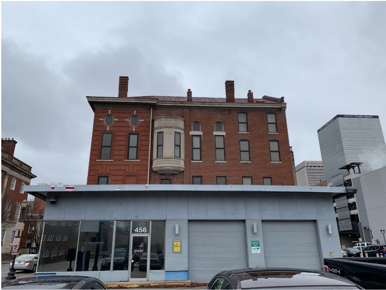
Figure 4. View looking at west at the East elevation.
