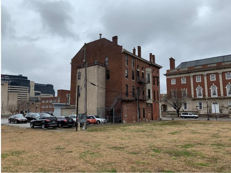
Figure 6. View looking at southeast at the West and North elevations.
