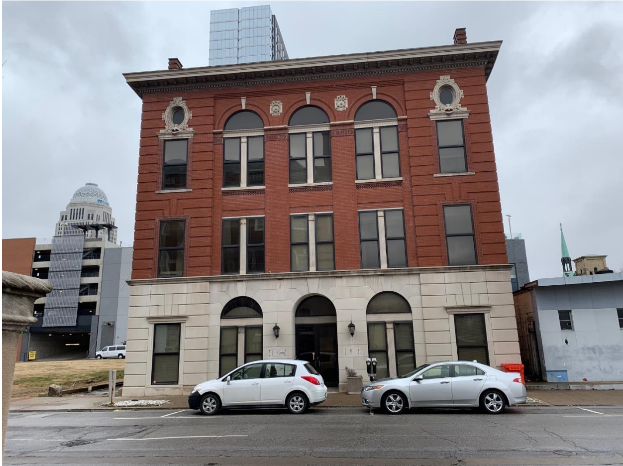
Figure 2. View looking North at the primary (South) facade.
