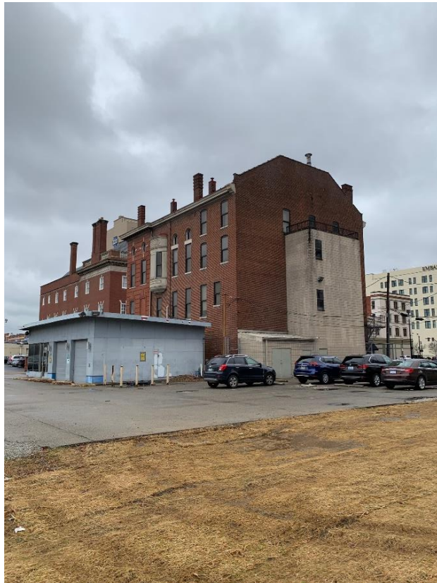
Figure 7. View looking at southwest at the East and North elevations.
