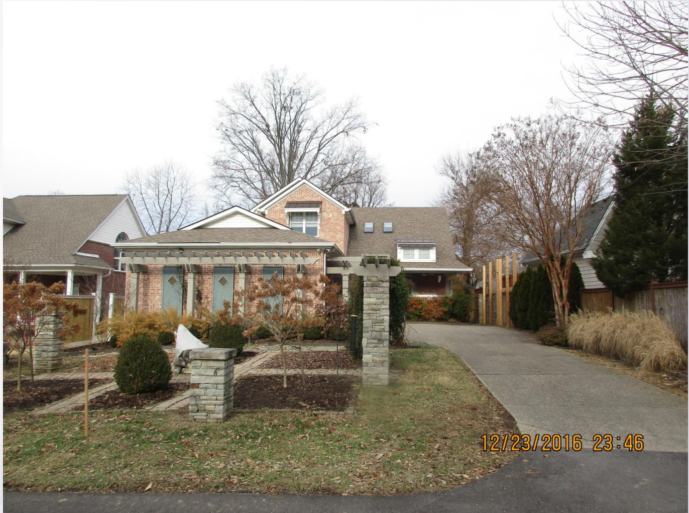
Subject Site, looking NW from Kennison Court.
