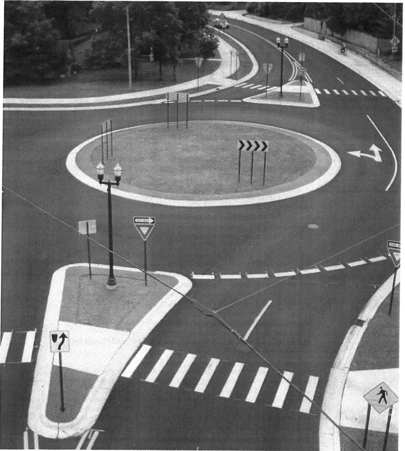
Figure 3.10 - The photo above represents a roundabout in a suburban setting that allows smooth traffic flow and clear pedestrian connectivity in Okemos, Michigan.
