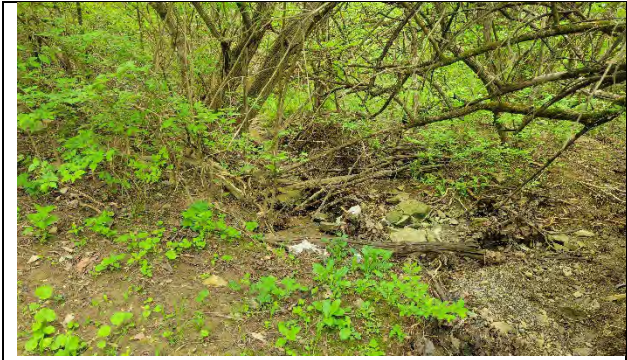
Photo 31: View of culvert and drainage swale (Slope Area 12).
