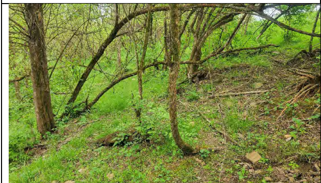
Photo 29: View of bowed trees and slope (Slope Area 11).
