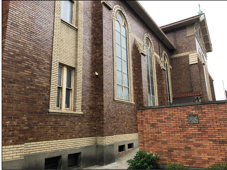
Figure 4. North elevation of Building 1, looking southwest.
