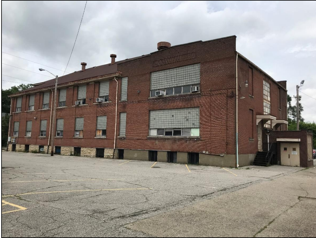
Figure 13. South elevation of Building 3, looking northwest.
