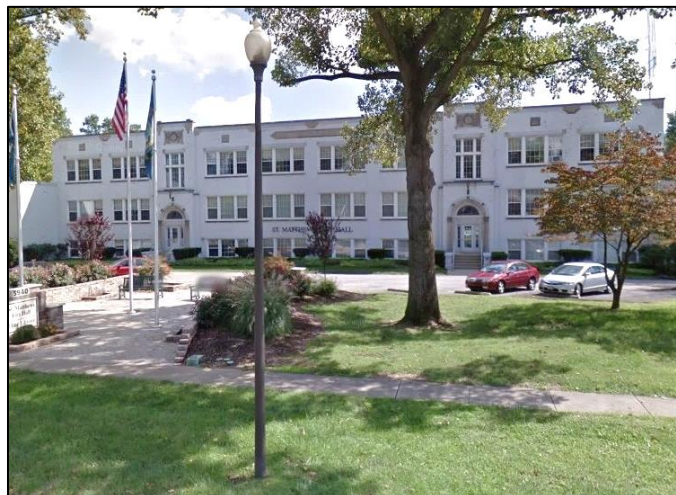
Figure 54. Greathouse School, 3940 Grandview Avenue (Google)
