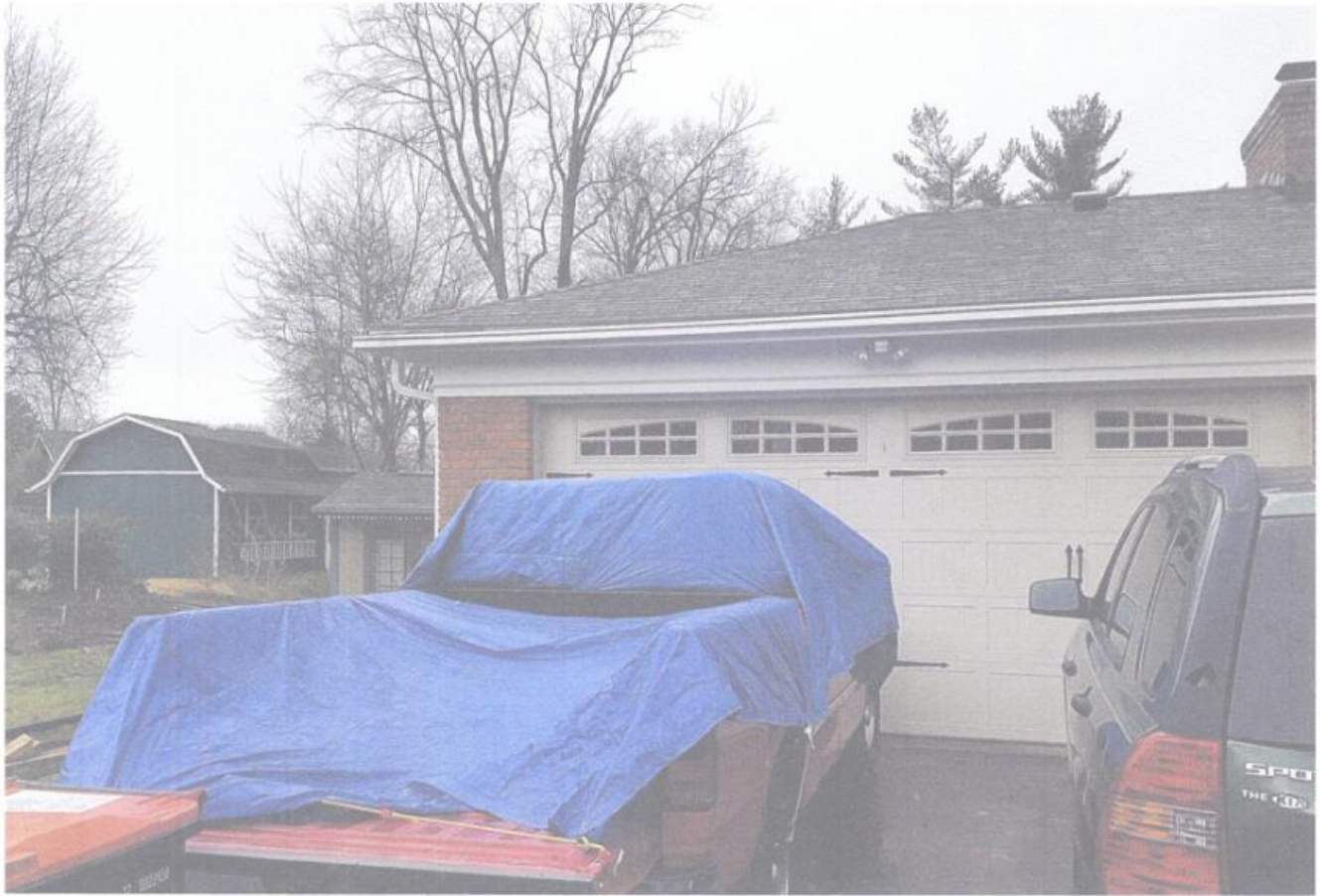
The existing garage.
