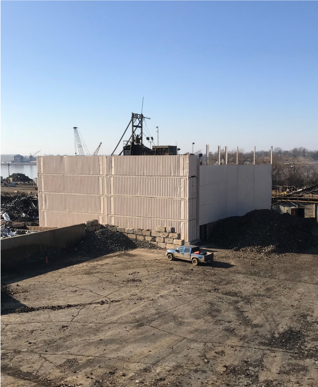
Current Noise Barrier Wall – Constructed in 2019
