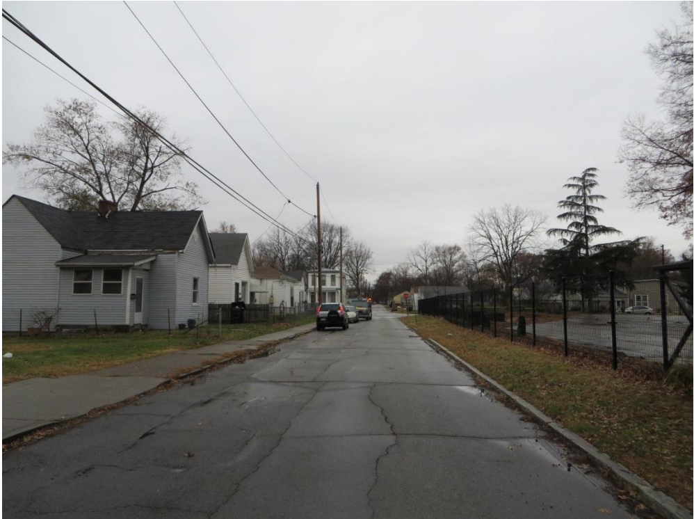
Looking West up Pflanz Avenue toward 35 th Street
