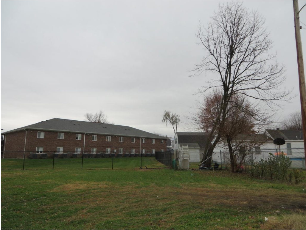
Existing multi-family residential property to the South
