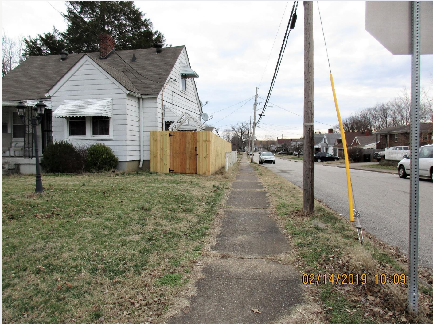
Ottawa Avenue Frontage from S. 1st Street
