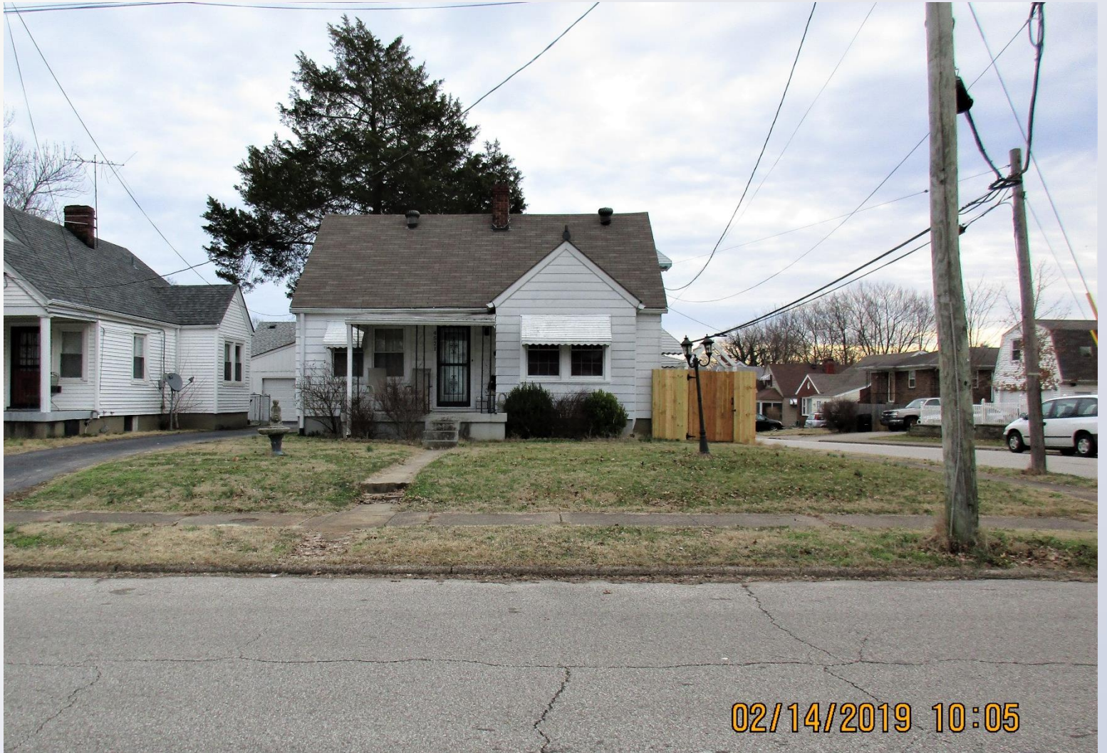
S. 1st Street Frontage
