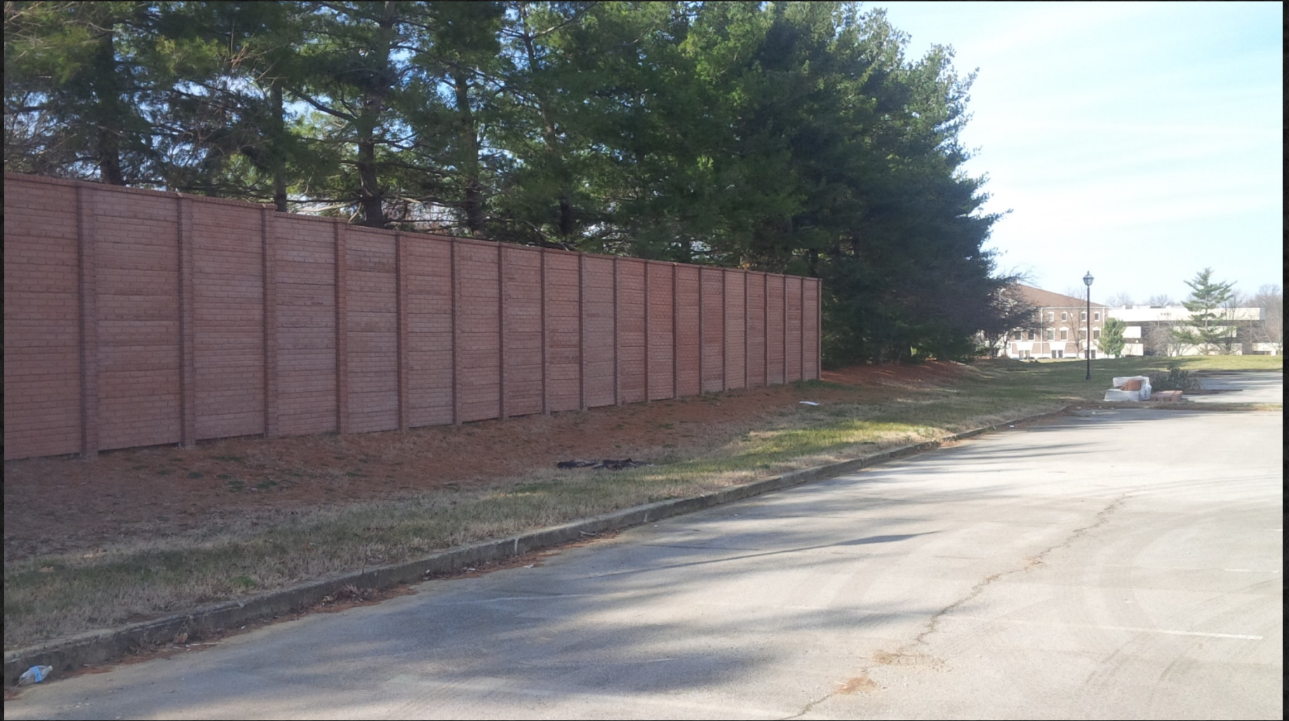
Proposed 8 ft masonry wall to be located along the north property line
