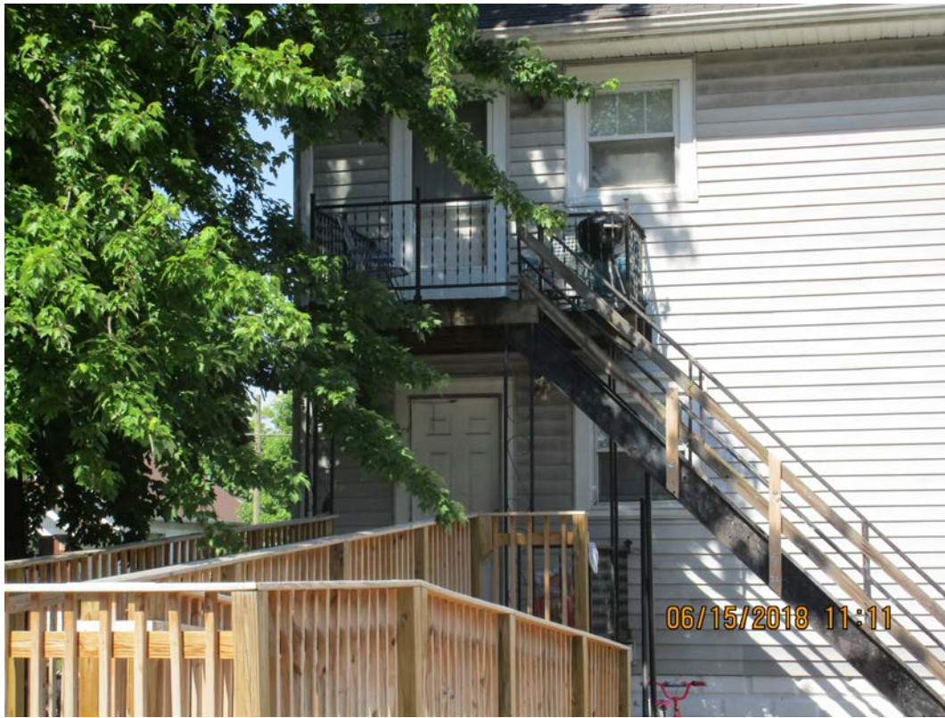
6. Rear stairs and entrances
