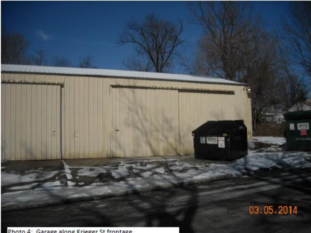
Photo 4: Garage along Krieger St frontage
