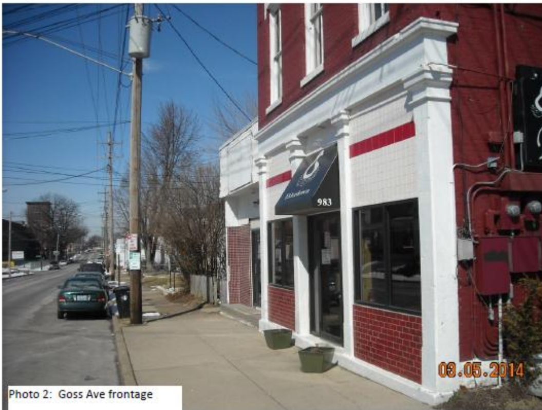
Goss Ave frontage showing front facade at street level and existing on-street parking restrictions.
