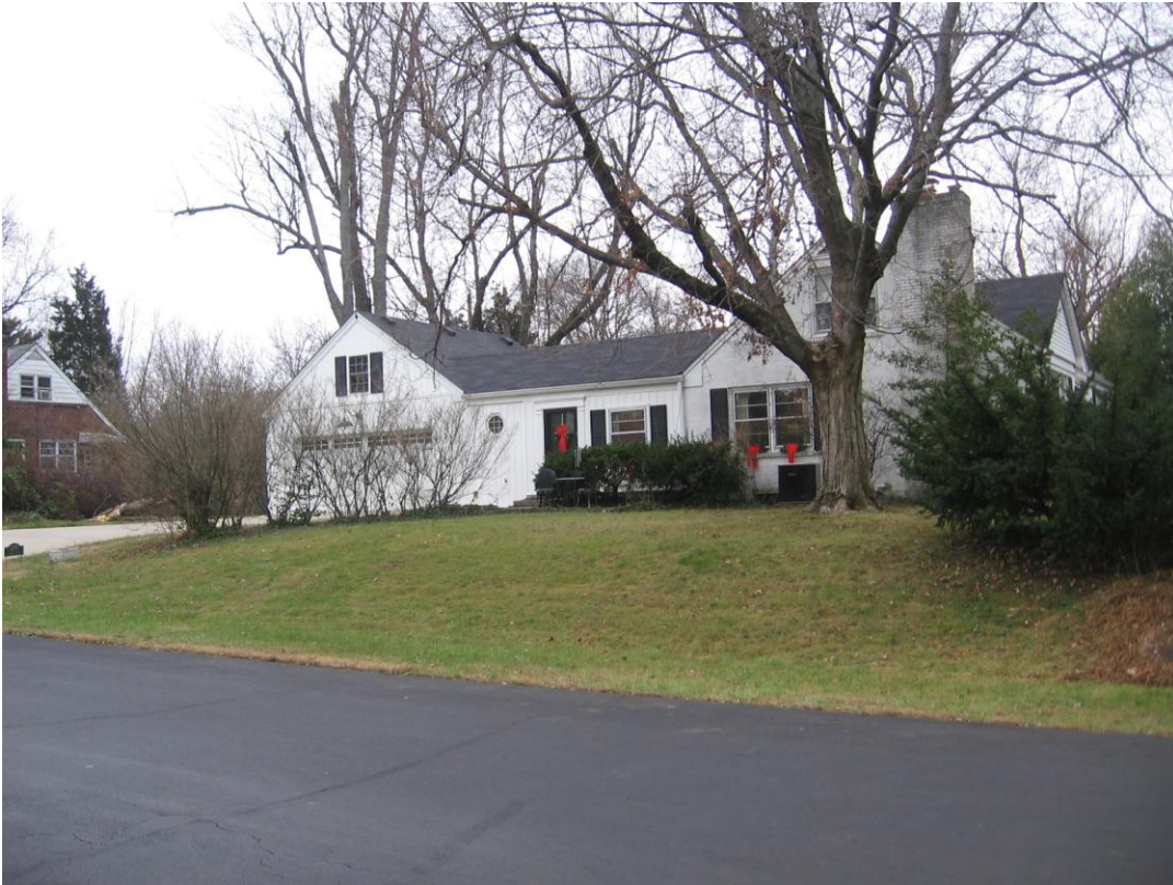
Looking west at the house directly across Miles Road
